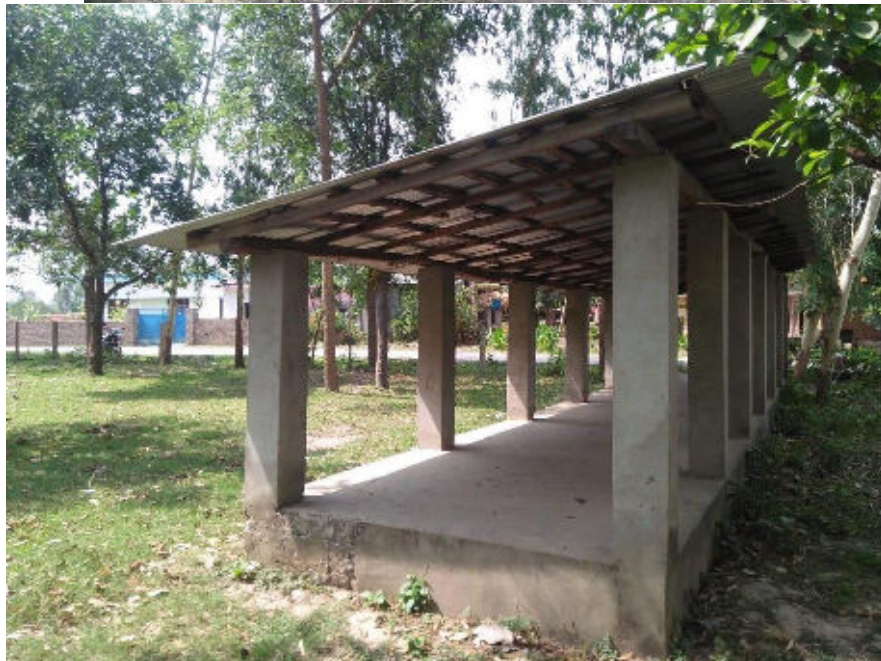
The shed to be dismantled
