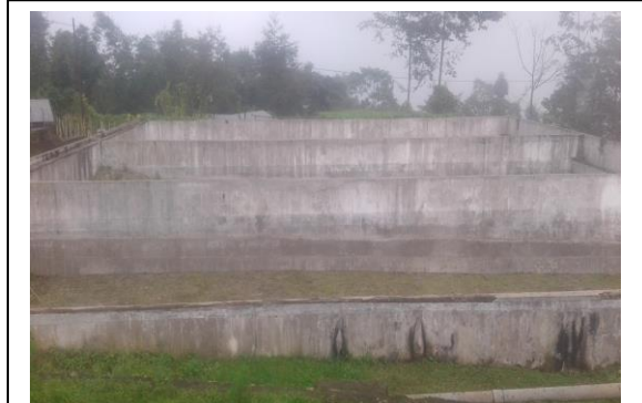
4. Non-functioning Existing Slow Sand Filter
