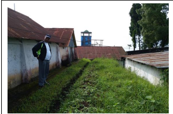
1. Existing RVT to be demolished
