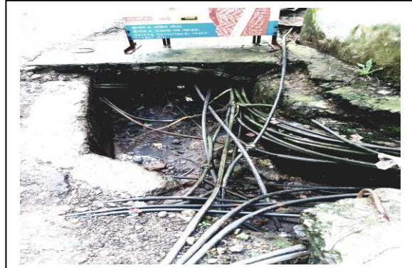
2. Existing condition of distribution pipelines
