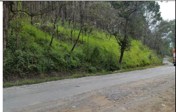
Access Road to the project location
