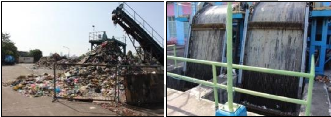
Figure 3: Solid wastes screen installed in Vitas Pump Station (left) and solid wastes collected by the trash rakes (right)
