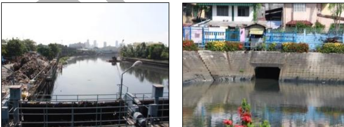
Figure 17: Intake of Vitas Pumping Station (left) and Balut PS (right)
