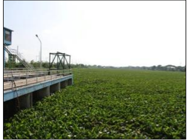
Figure 14: Labasan Pumping Station: trash trap (left) and water hyacinth accumulating in the retention pond (right)
