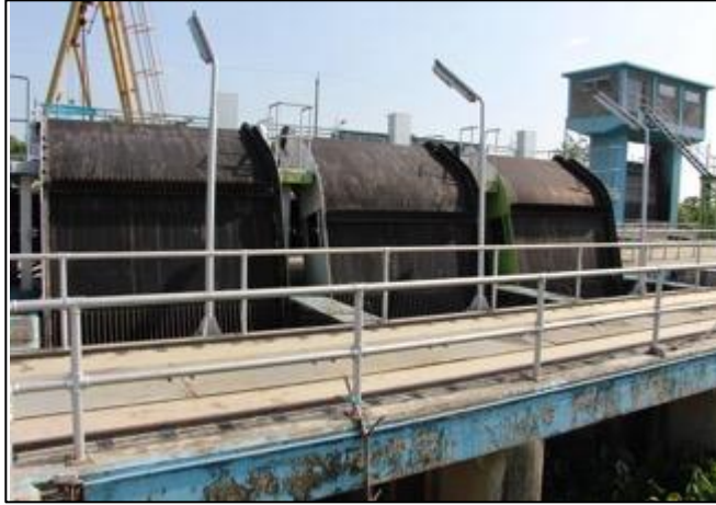
Figure 14: Labasan Pumping Station: trash trap (left) and water hyacinth accumulating in the retention pond (right)
