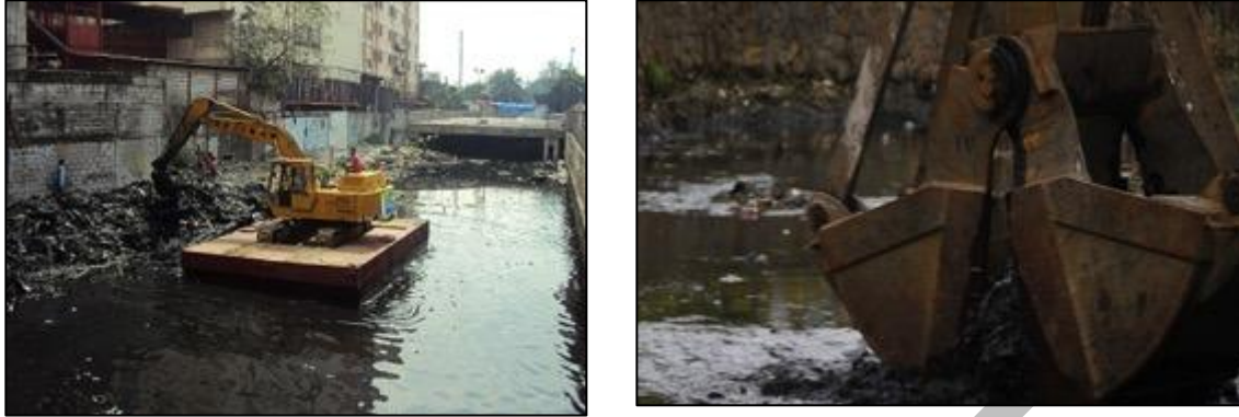
Figure 15: Dredging of narrow esteros leading to pumping stations (Source: www.aarcon builders.com & www.abs-cbn.com)
