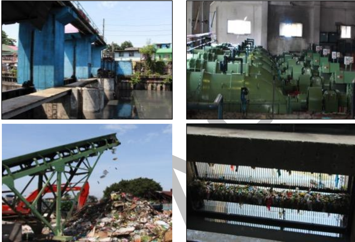
Figure 12: Tripa de Gallina Pump Station (above) and solid wastes collected (below)
