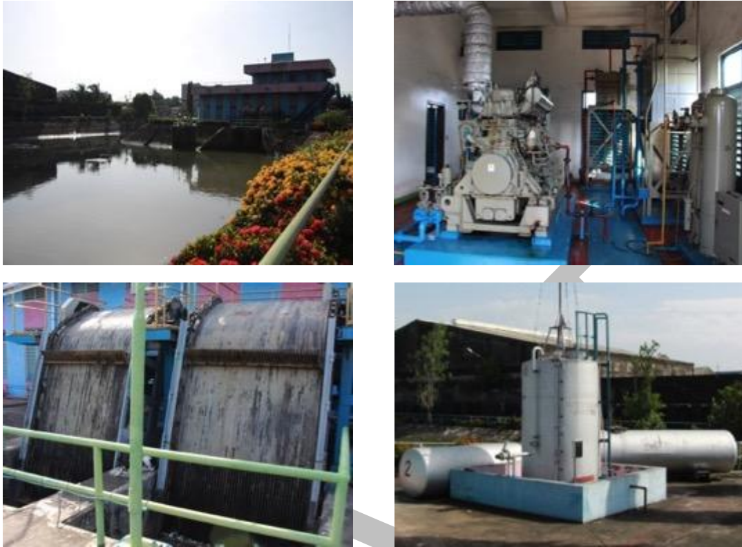
Figure 8: Balut Pumps Stations, Pump House, Solid Waste Collector and Diesel Storage Tank (clockwise)
