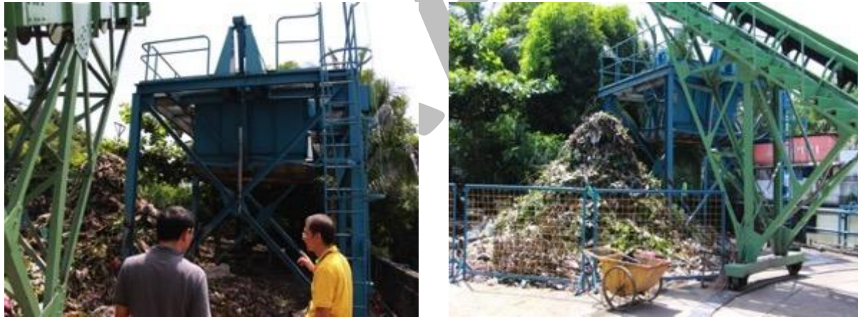
Figure 10: Solid waste collection at Paco Pumping Station
