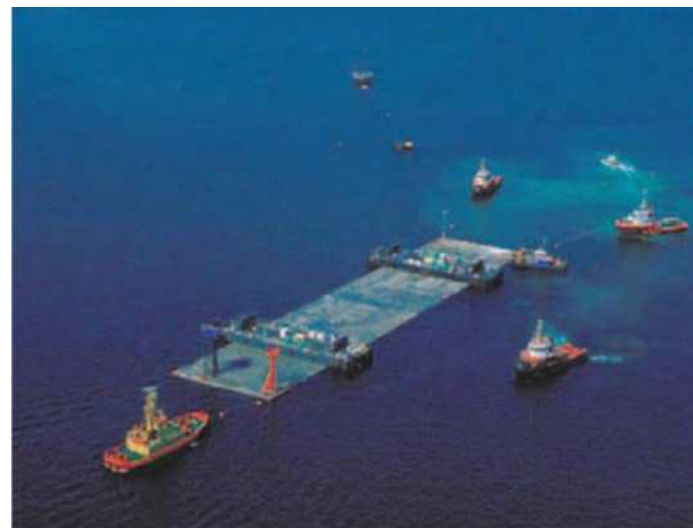
Figure 8.9. Bedding of the concrete tunnel element on the site.
