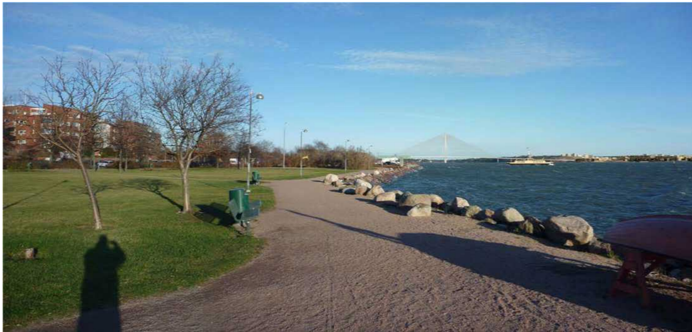
Figure 9.48. The Kruunu Mountains bridge from the north-eastern beaches of the Herttoniemenranta Tuorinniemi. Visual picture of the Visual Analysis Study (Draft), WSP Finland
