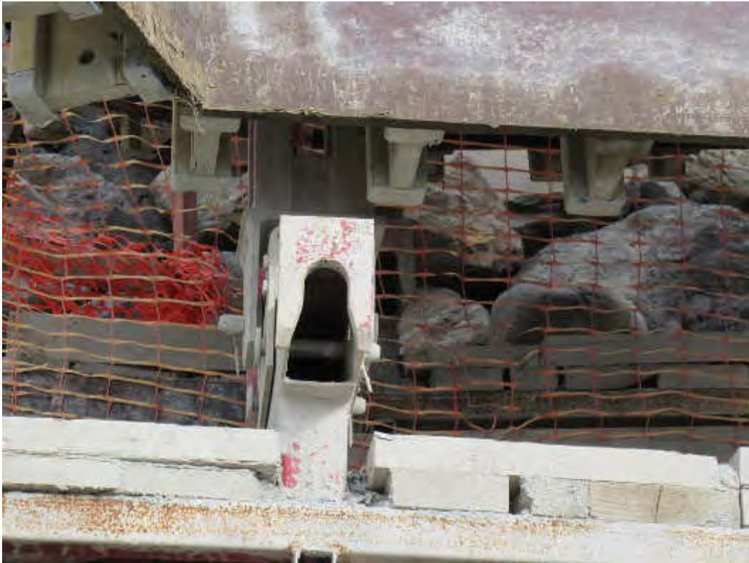
Photograph 8 Close up of slot mechanism that receives the tapered locking pin
