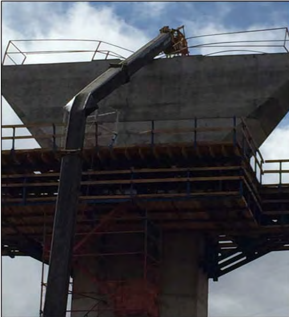
Photograph 2 Crane mast buckled
