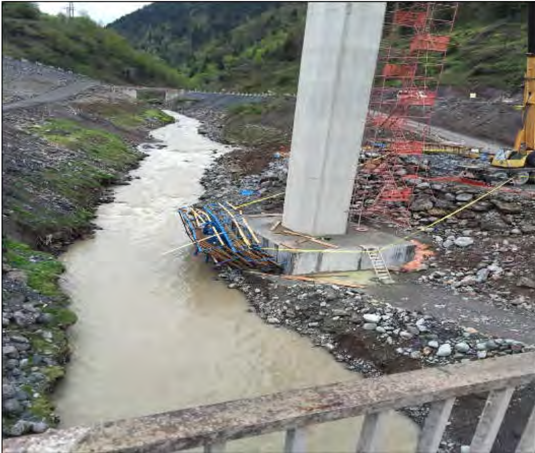
Photograph 4 Fallen work platform
