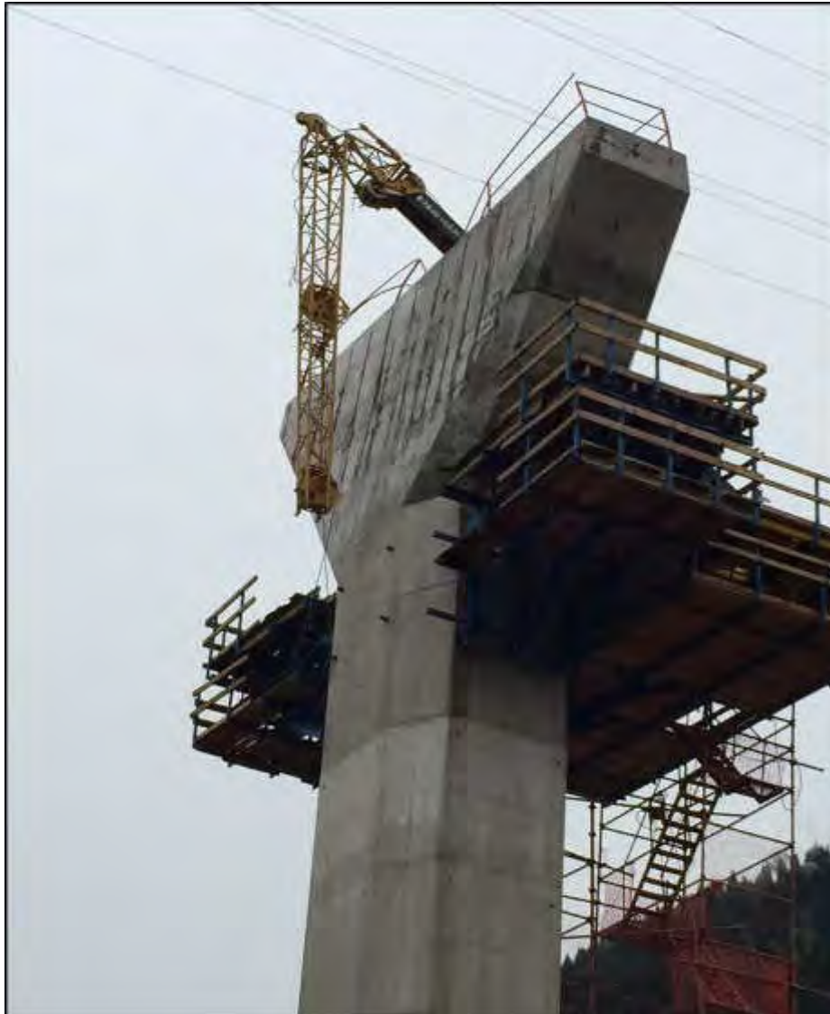
Photograph 3 Fly-jib buckled, showing two sections of fly-jib were used
