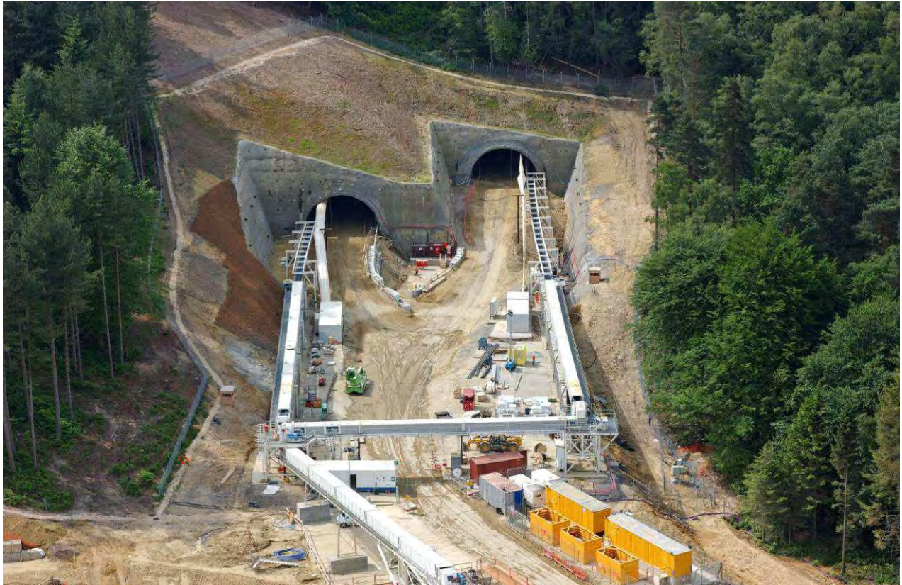
Figure 2.8: Example of Tunnel and Portal Construction
