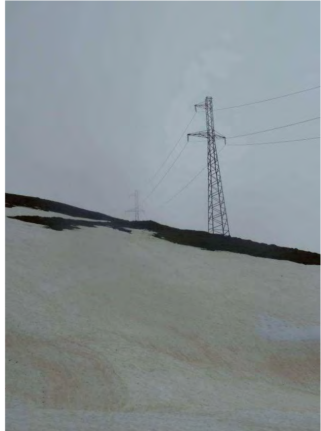
Figure 2.13: Existing 110 kV transmission line
