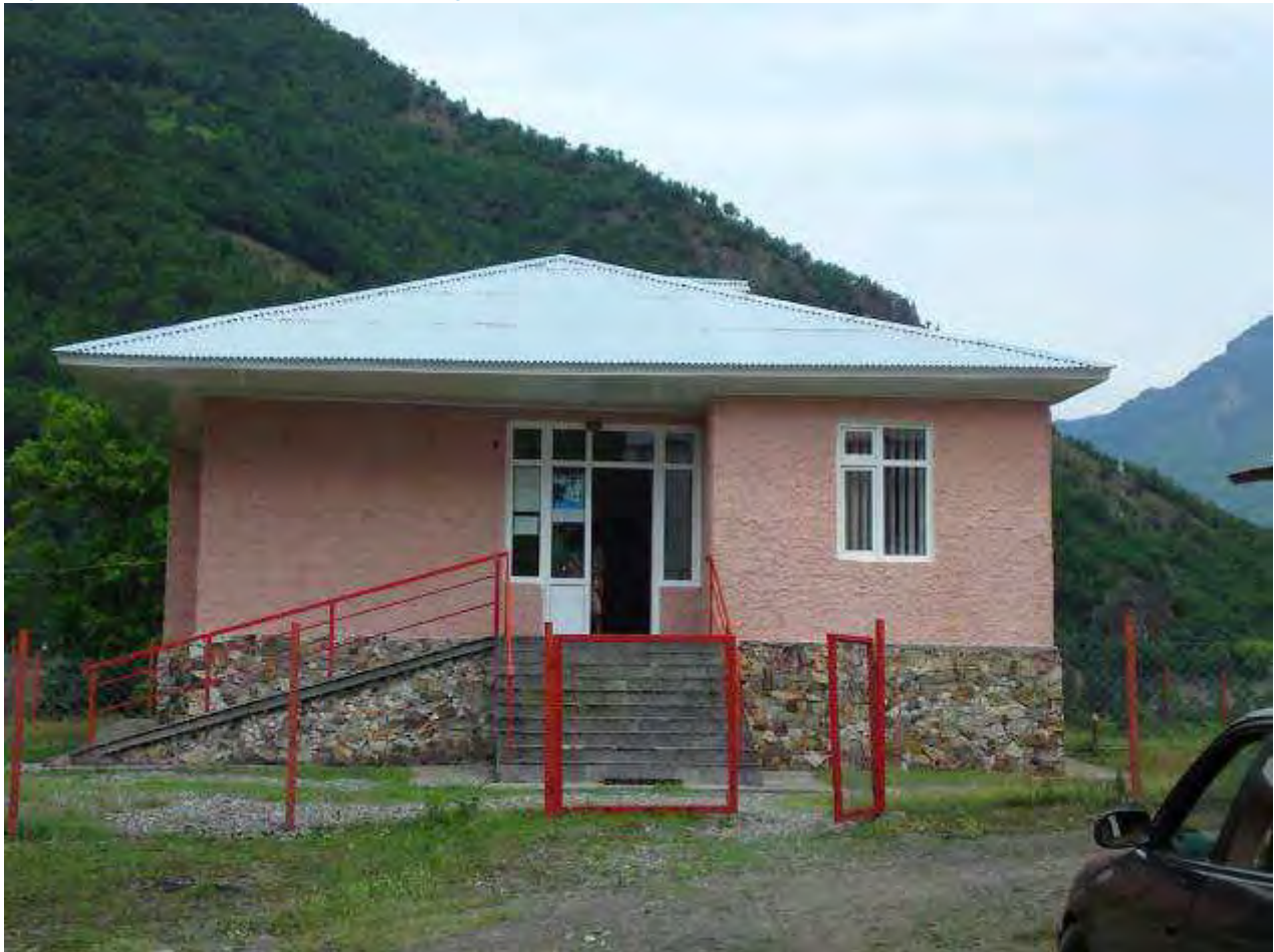
Figure 7.3: Health centre in Zamleti village
