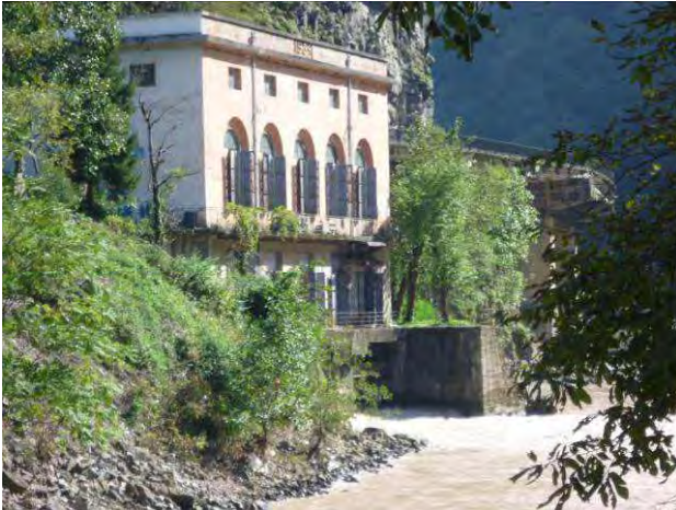
Figure 2.9: Existing Asti HPP Surface Powerhouse
