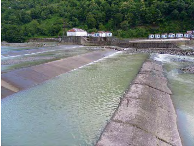
Atsi HPP Weir and Intake Facilities
