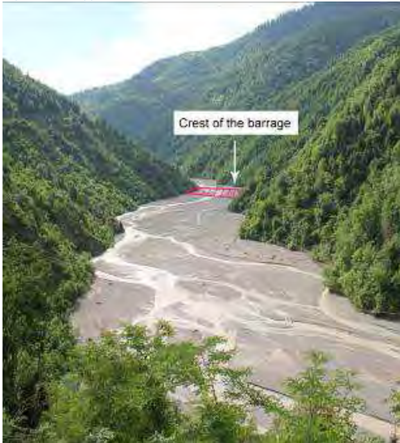
Figure 18.7: Approximate line of crest of Skhalta dam
