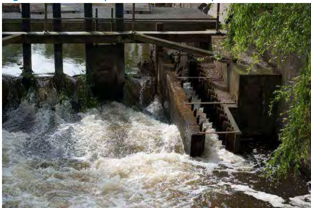
Figure 2.6: Examples of different fish pass structures
