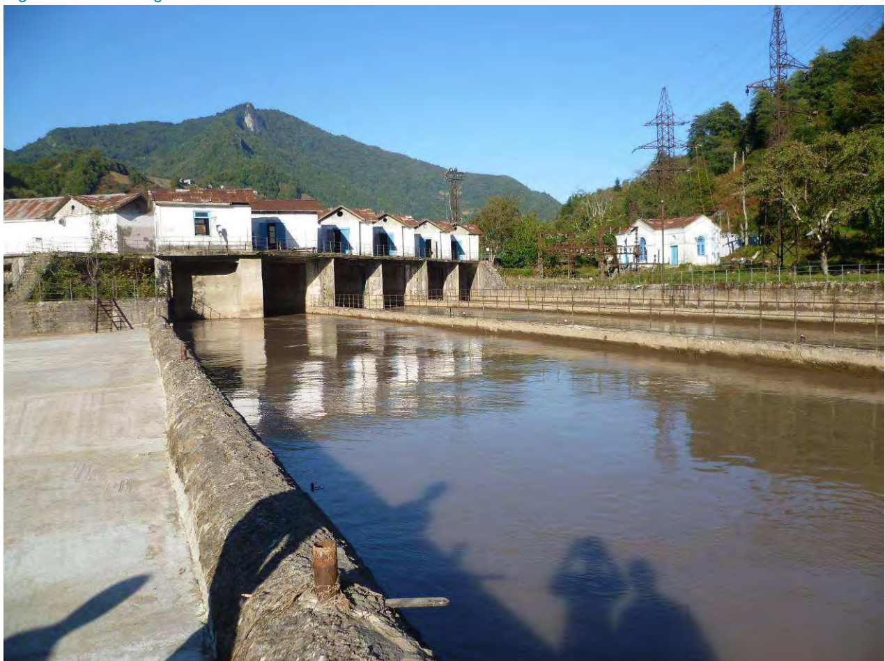
Figure 2.5: Existing Asti HPP Sediment Basin
