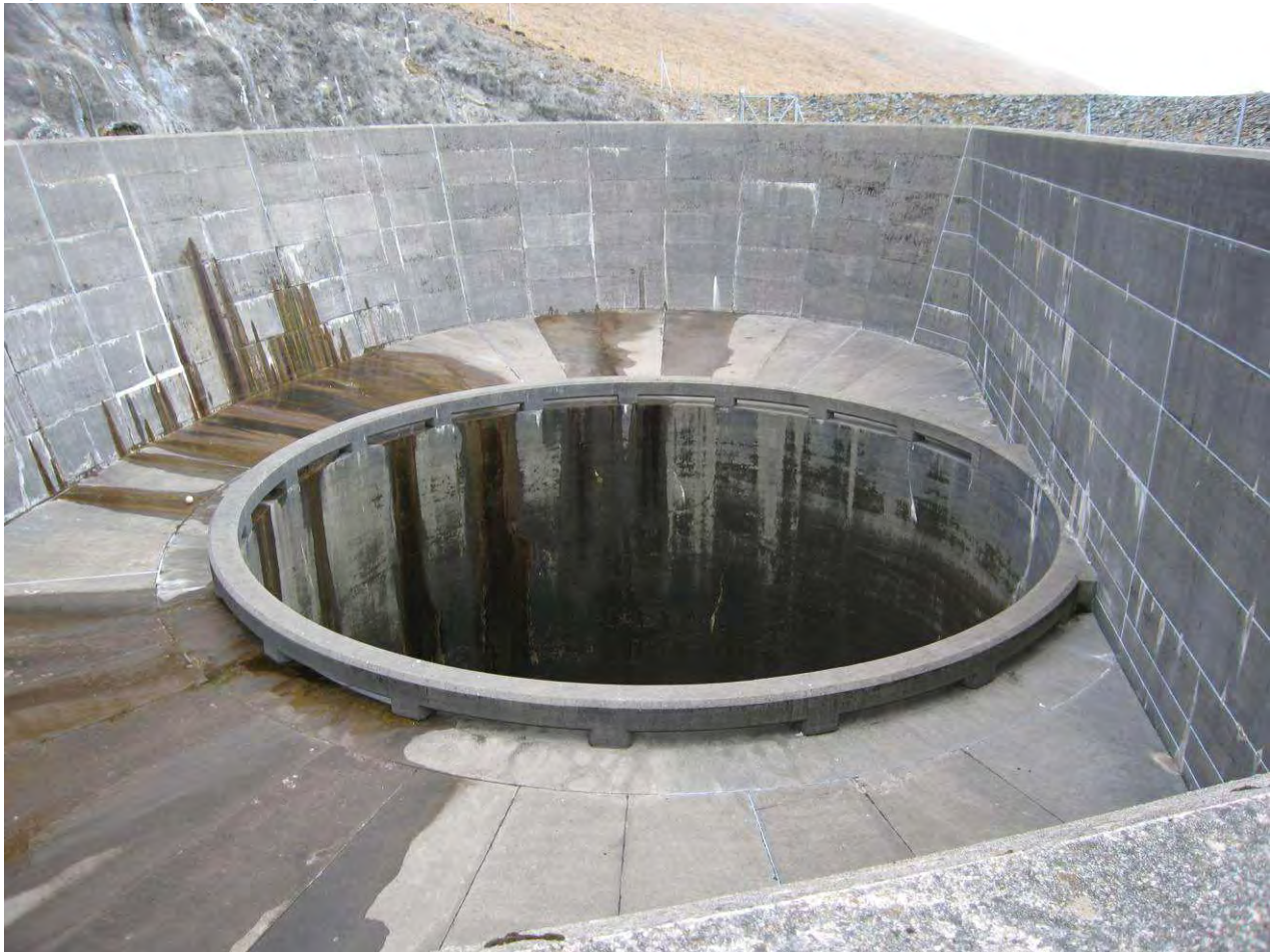
Figure 2.7: Example of surge shaft
