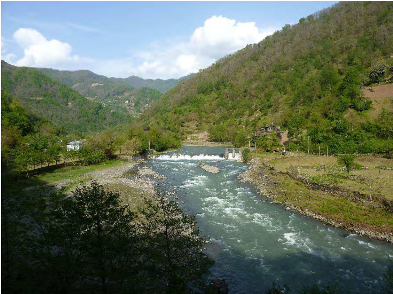
Figure 2.4: Existing Machakhlistsqali HPP Concrete Weir
