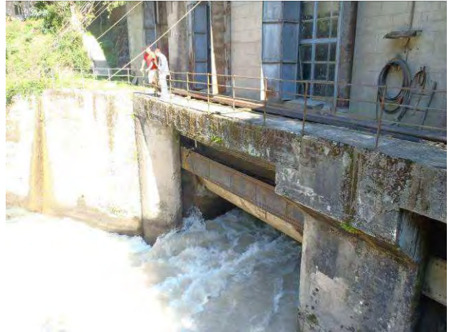
Figure 2.10: Existing Asti HPP Tailrace
