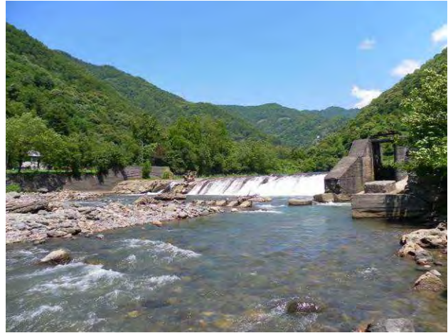
Existing Machakhlistsqali HPP
