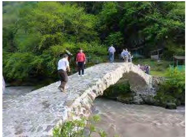
Figure 18.5: View of historic bridge near proposed Khertvisi Reservoir
