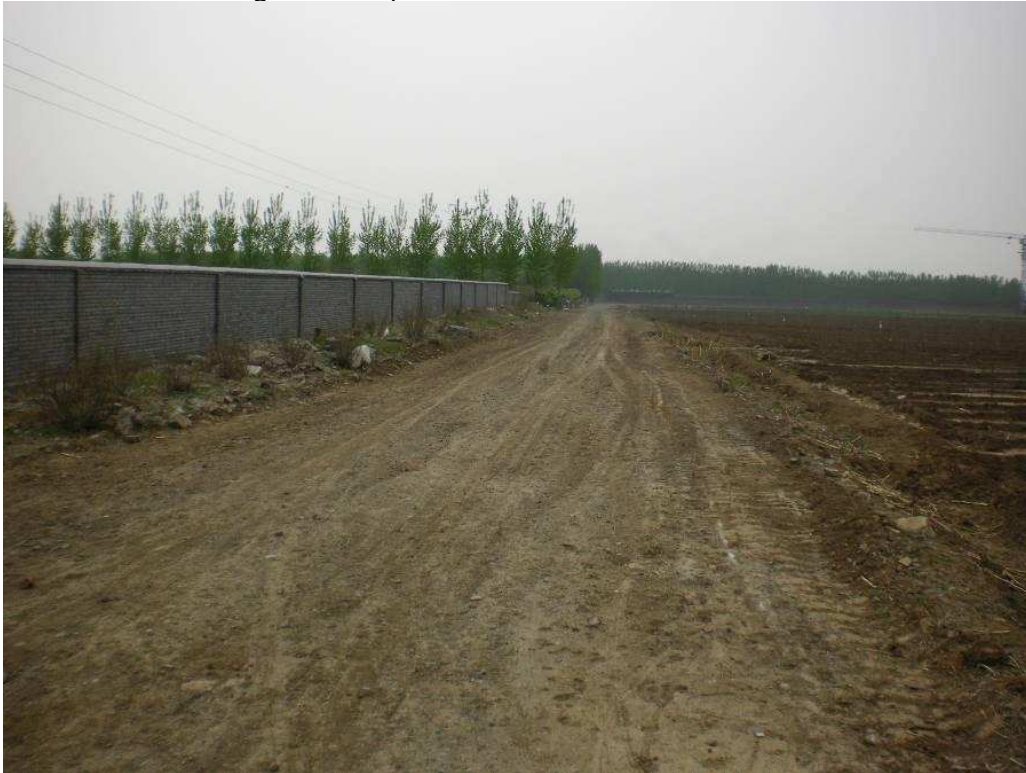
Figure 3-Acquired Land for the Access Road
