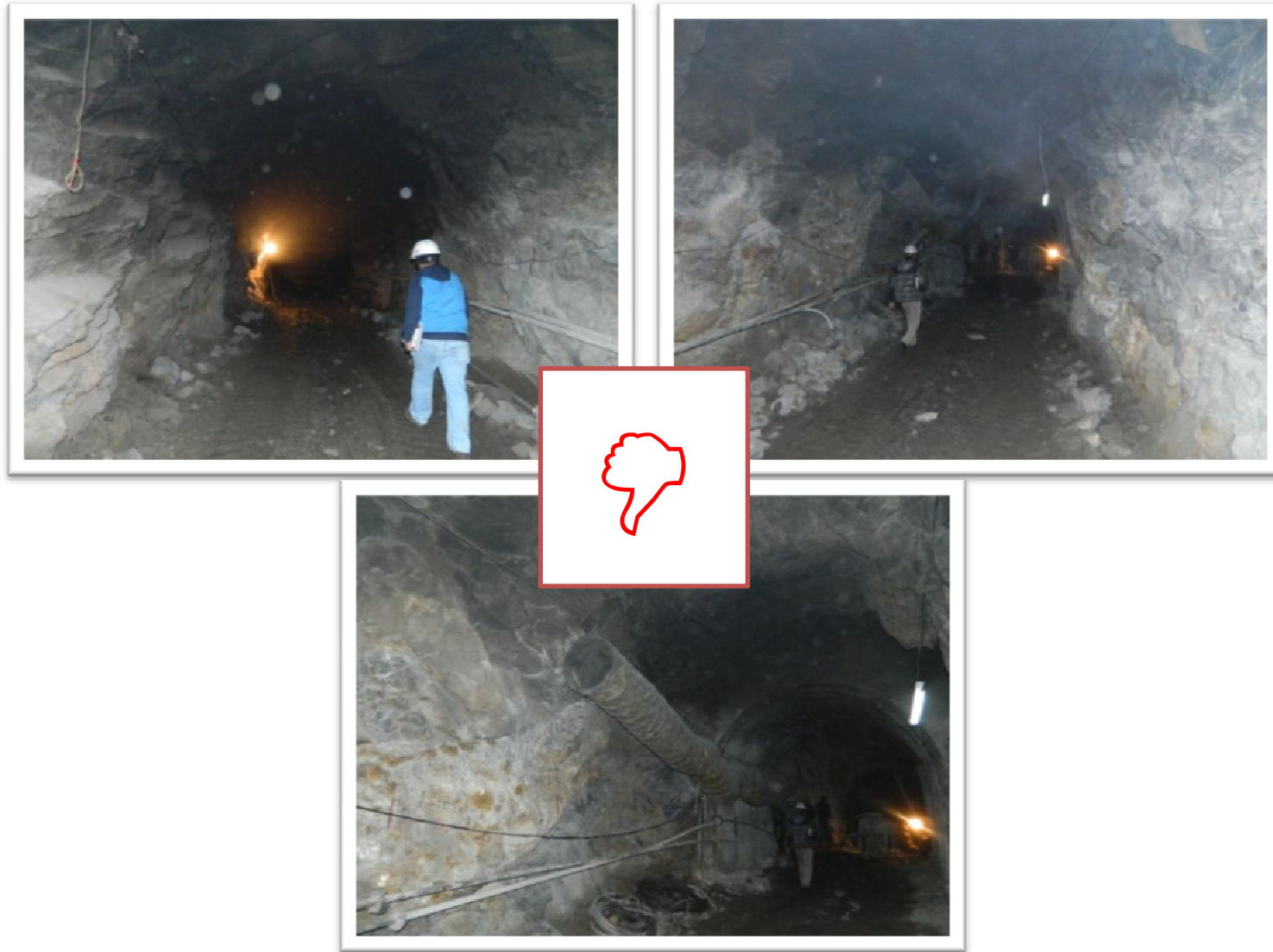
Poor ventilation and illumination in underground works i.e. Adit-4
