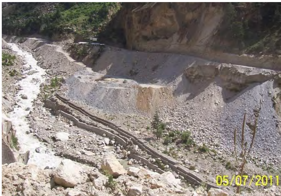
Figure 5-2: Muck dumping site along Tidong River with retention wall
