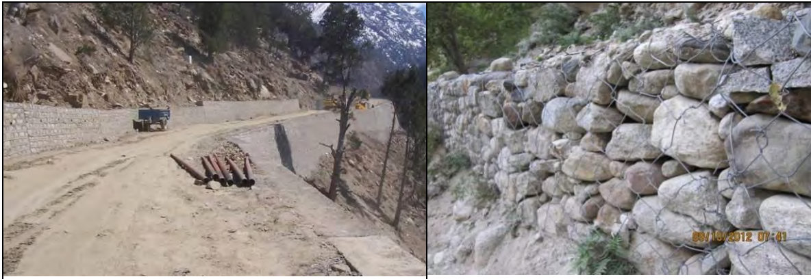
Figure 5-1: Retention wall provided at power house site (left) and bank protection at Lambar (right)
