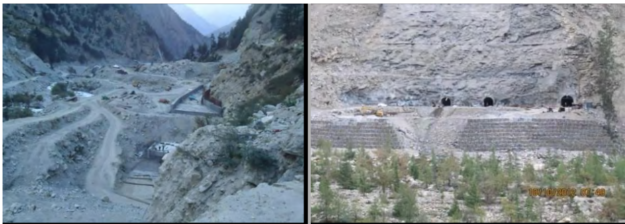
Figure 3-5: Photographs from site
