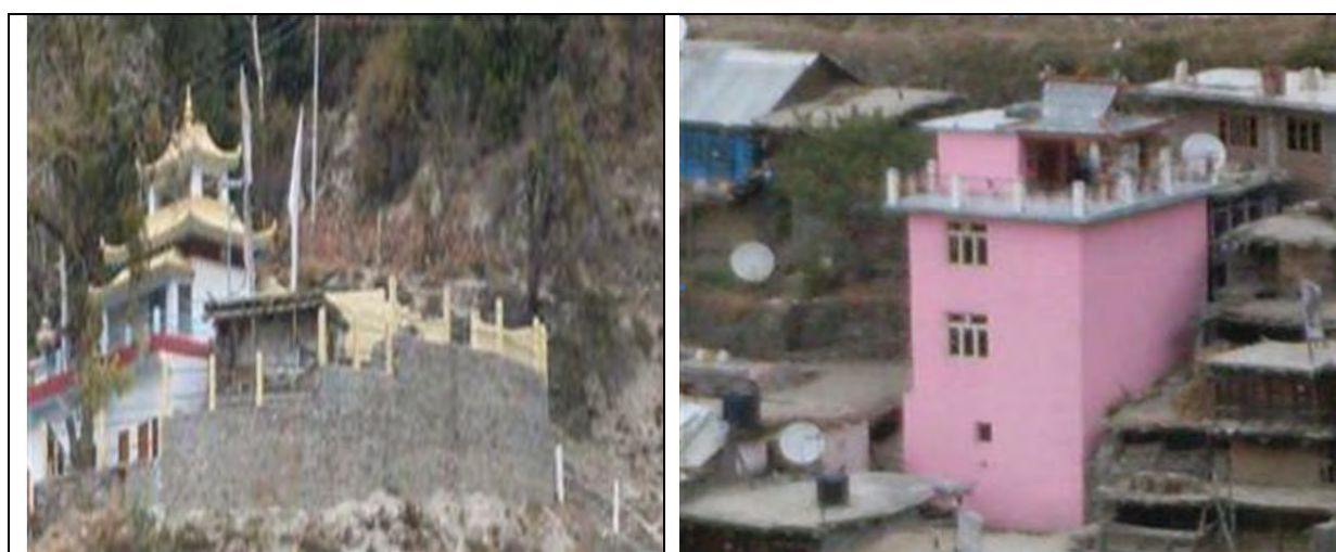
Retaining Wall at Temple (Left) and Community Hall with Temple (Right) in Moorang under LADA
