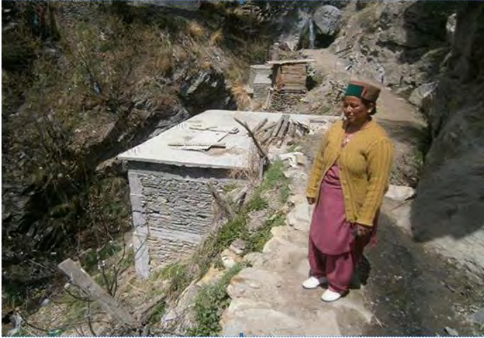
Community Septic Tank completed at Ghatla in Thangi Panchayat
