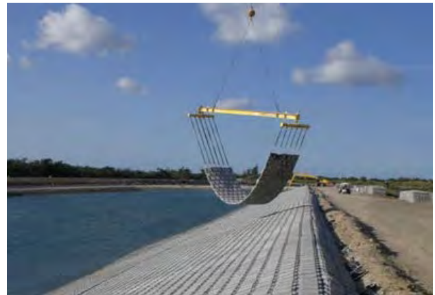
Figure 2.8: Closed Concrete Block Lining
