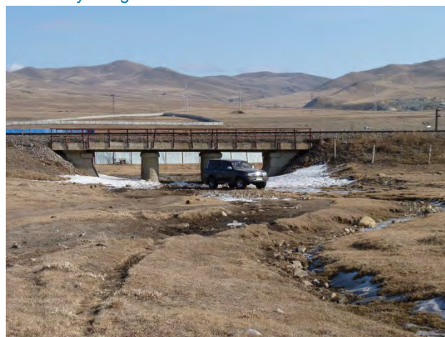
Photo 9.10: Northwest Tributary Immediately Upstream of Railway Bridge
