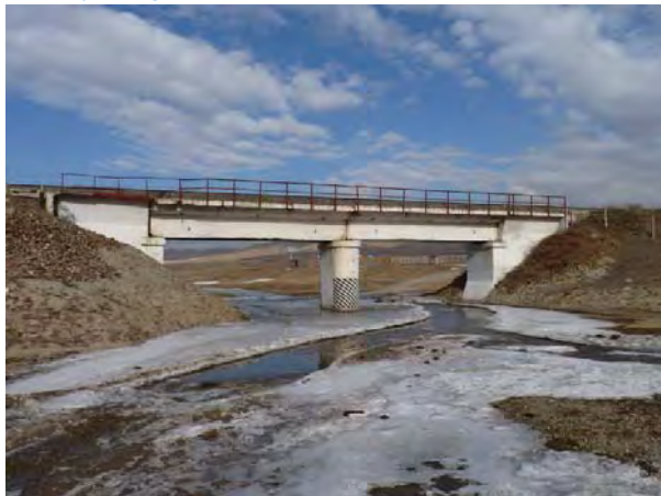
Photo 9.1: Khuliin River Immediately Upstream of Railway Bridge
