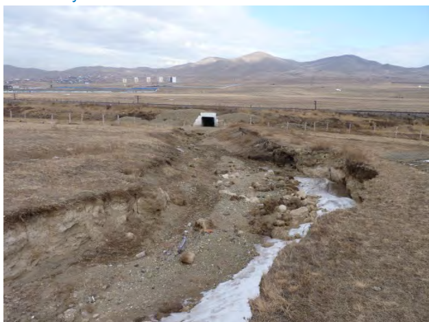
Photo 9.11: Southwest Tributary Immediately Upstream of Railway Box Culvert
