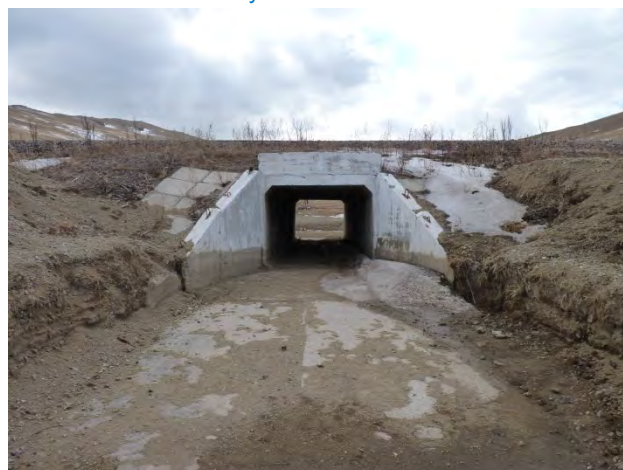
Photo 9.12: Southwest Tributary Immediately Downstream of Railway Box Culvert
