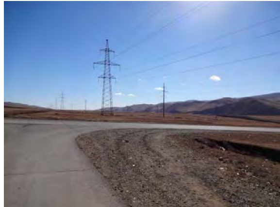
Figure 14.5: View from the Happy Valley development looking south along the valley towards the site.
