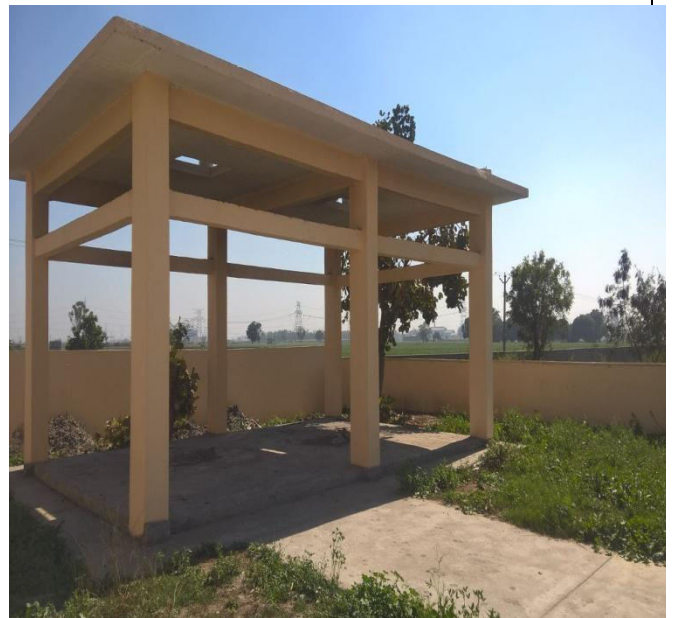
CONSTRUCTION OF SHED AT SHAMSHAN GHAT
