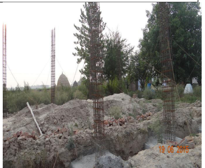
CONSTRUCTION OF COMMUNITY CENTRE
