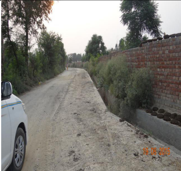
CONSTRUCTION OF INTERLOCKING PATH WITHIN THE VILLAGE
