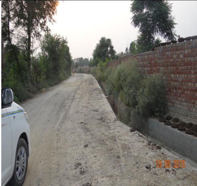
CONSTRUCTION OF INTERLOCKING PATH WITHIN THE VILLAGE
