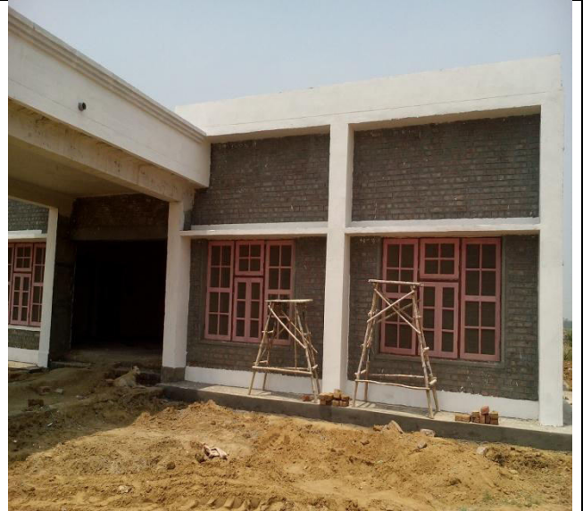
CONSTRUCTION OF COMMUNITY CENTRE
