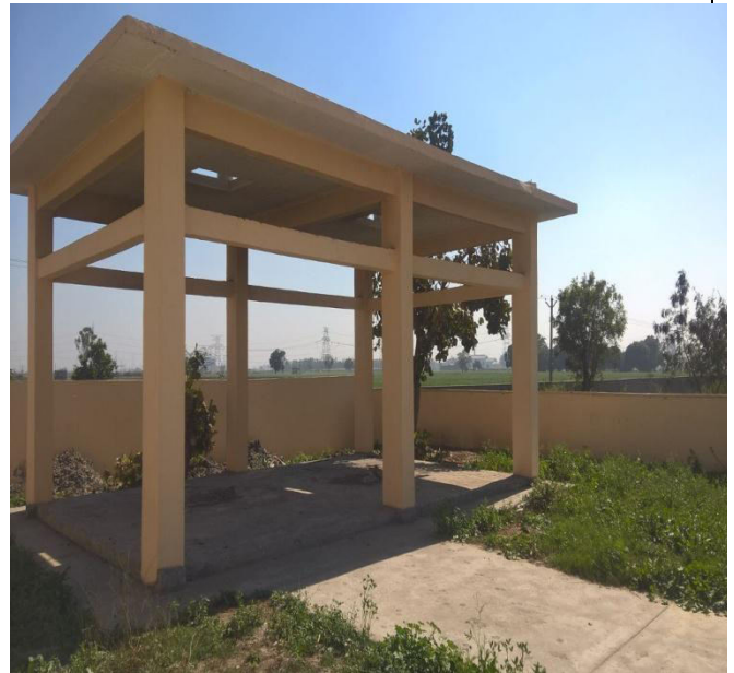
CONSTRUCTION OF SHED AT SHAMSHAN GHAT
