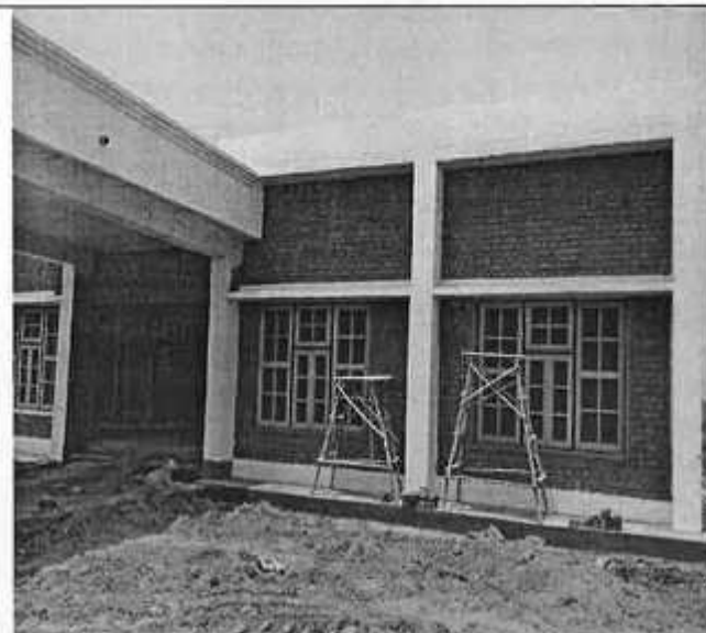
CONSTRUCTION OF COMMUNITY CENTRE
