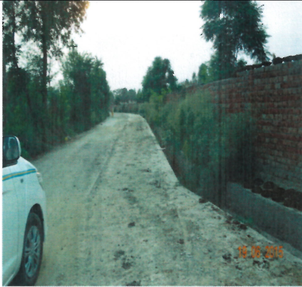
CONSTRUCTION OF INTERLOCKING PATH WITHIN THE VILLAGE
