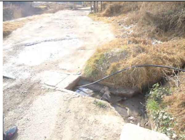
Clogged drains with no further connection for exit
