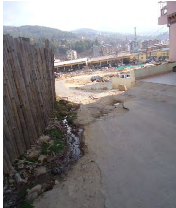
Drain flowing across the road
