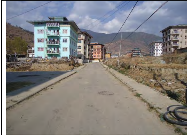
Road condition at Babesa
