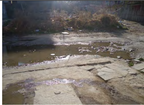
Water logging on the road at Changzamtog
