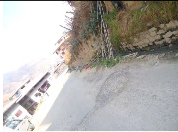
Road stretch at Changzamtog
