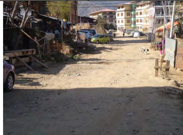
Road condition at Kala Bazar area
