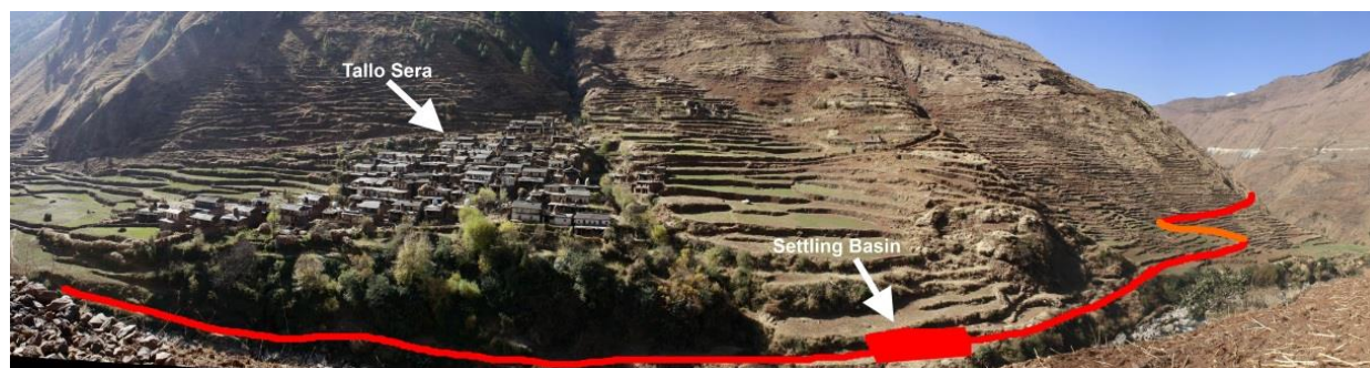
Figure 5.1: Sani Veri Headrace Canal (initial section) and Settling Basin
