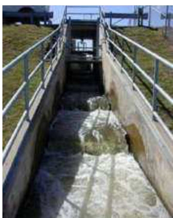
Figure 12.2: Pool-and-Weir Fishway
