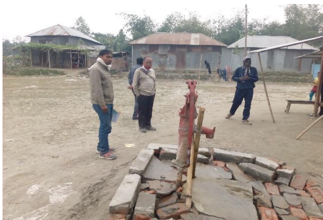
8. Broken protection of tube well
