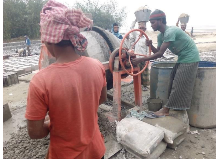
5. Concrete mixture machine is driven without safety equipment
