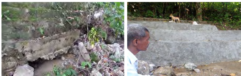
Figure 5.1 Repair of "Ambar" Irrigation body at Pardamean Nainggolan village
