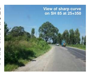
234. Thus the section from Km 24+700 to Km 25+756 (existing) has 4 very poor horizontal curves within a short length. Hence, to improve safety of the road users, geometric improvement in form of realignment has been proposed for a length of 900 m from Km 24+700 to Km 25+600.
