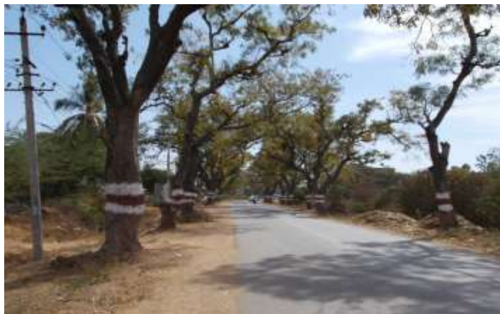
View of Trees along Project Road
