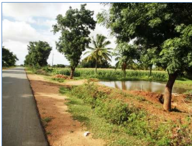
Partially Affected Water Storage Area at Ch. Km 142+800 at Devihala Village
