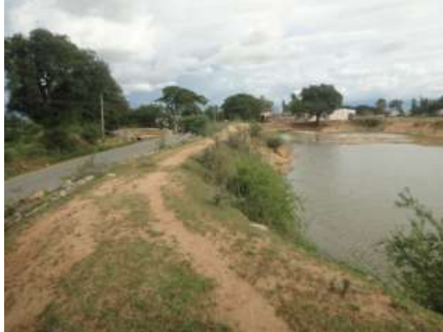
Pond at Ch. Km 144+600 on
