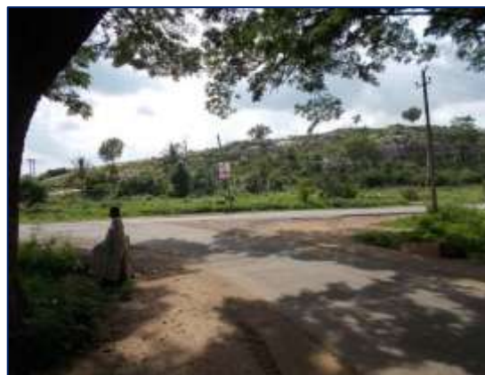
Take off point of Huliurudurga Bypass currently under construction in separate Package by KSHIP II
