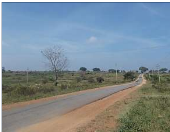
View of Project Road
