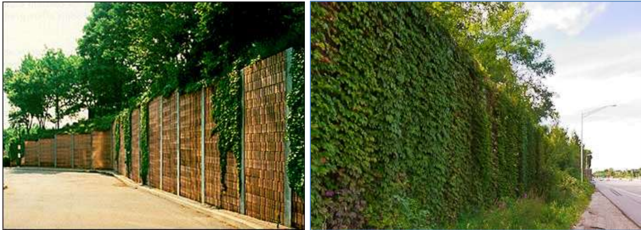
Figure 61 View of Solid Boundary Wall with Trees and Creepers
