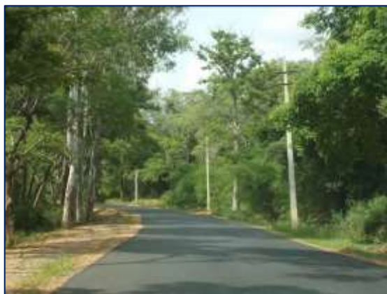
Project Road passing through Nagamangala Forest
