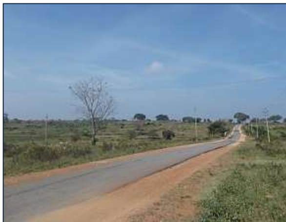
View of Project Road
