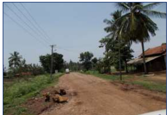
Project road badly damaged without pavement surface near Project Termination Point
