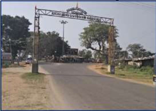
Figure 2: Start point of the Project on SH 85 at Ch. 51+815 in Magadi
