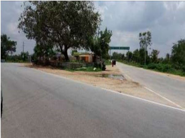
View of Junction of SH 99
