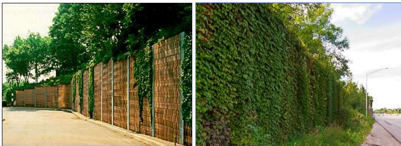
Figure 53: View of Solid Boundary Wall with Trees and Creepers
