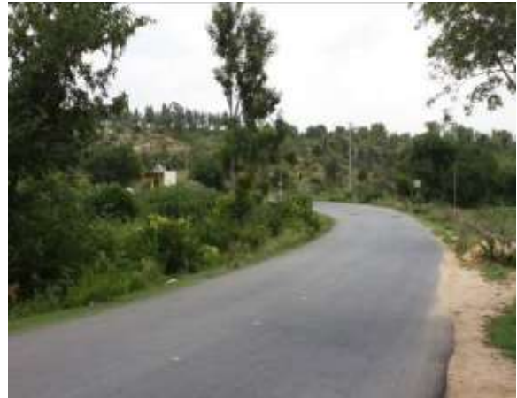
View of Sharp curve at Km 63+920
