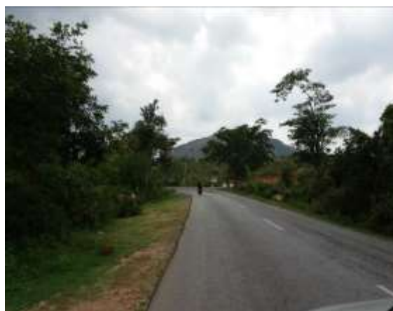
Blind curve at Km 75+600 with cross road
