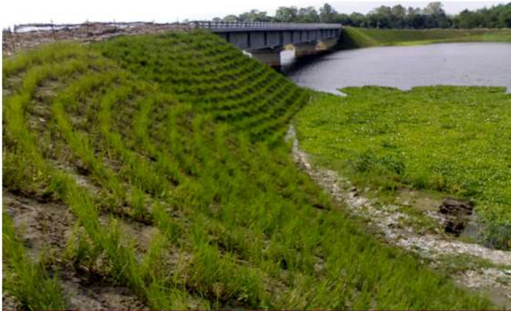
Vetiver Grass used for Slope Stabilization in Bridge ↑ & Road ↓ Embankment
