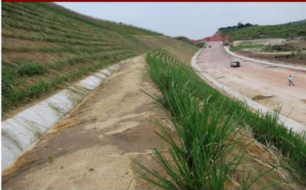
Vetiver Grass used for Slope Stabilization in Bridge ↑ & Road ↓ Embankment
