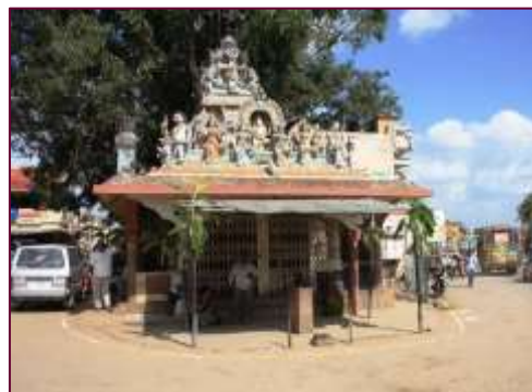
Vinayak Temple at Ch. Km. 49+985
