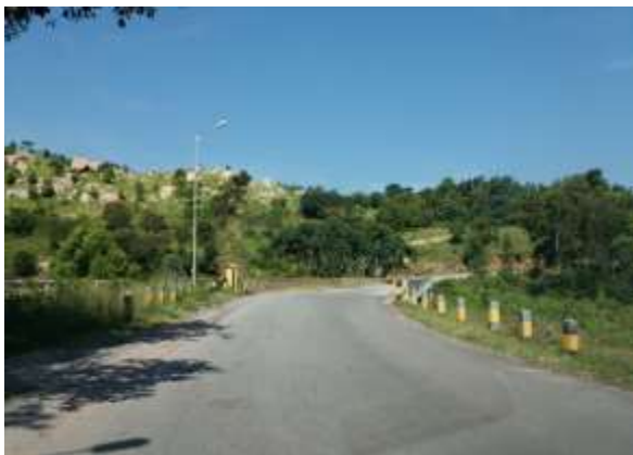
View of Sharp Curve at 34+200
