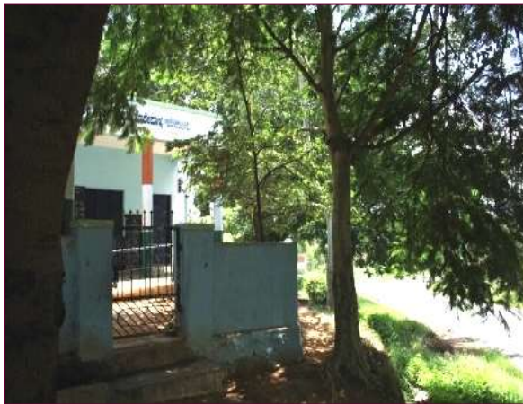
Photograph of Fully Affected Govt. Primary School at Ch. Km 42+080, Marlagondla
