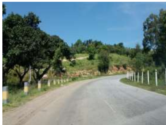
View of blind curve at Km 34+400 on bridge approach
