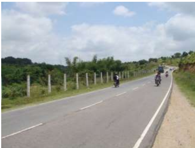
View of the Project Road near Ch km 32+000
