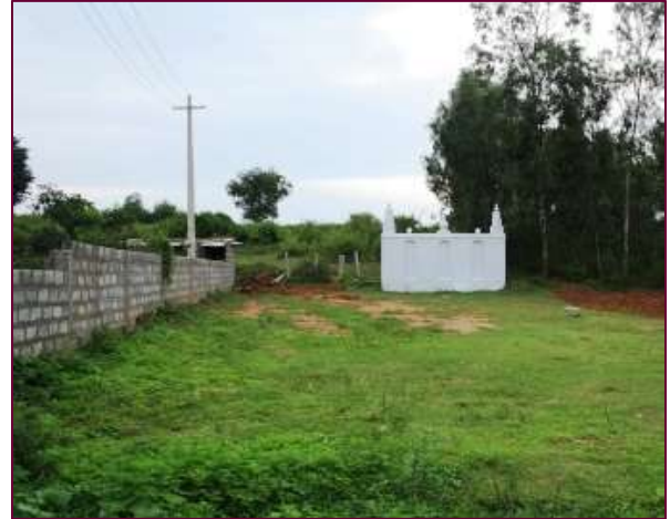
Idgah at Ch. Km 24+960
