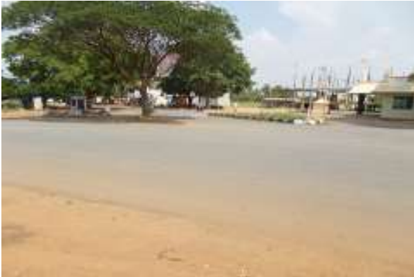
Figure 2: Start point of the Project at a junction with NH 234 and Km 47.450 on SH 82 near Chintamani
