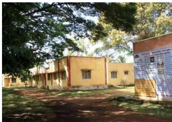
Primary Health Centre at Ch. Km 74+800 on RHS (Kamagere)
