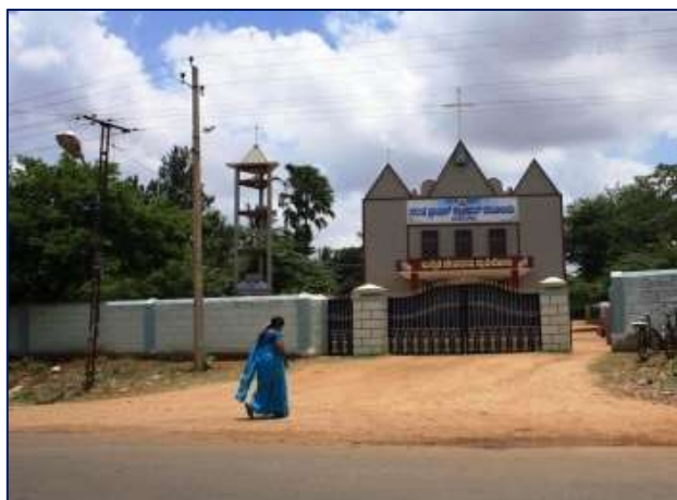
St. Francis Church at Ch. Km 76+000 on LHS (Konagarahalli Village)
