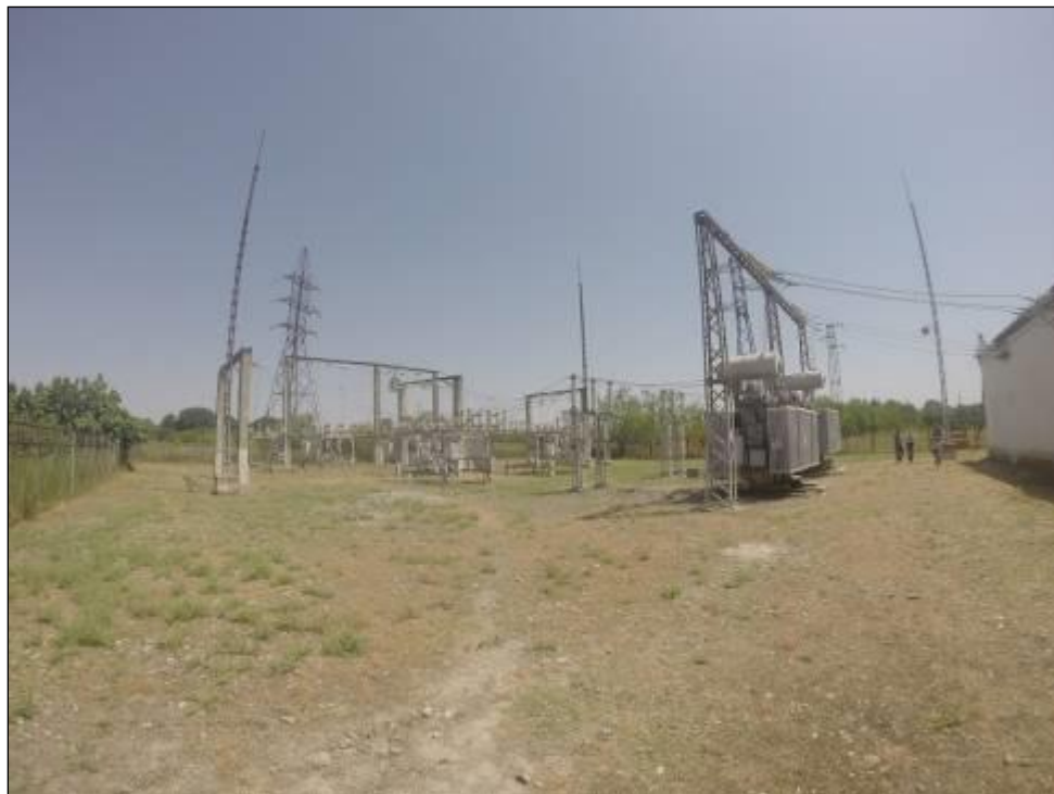
Existing 35 kV substation (Zardab) This is typical of substations that will be upgraded within the substation boundary
