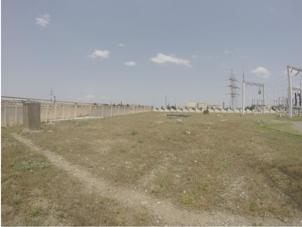
Proposed area for new 110 kV substation within the boundary of the existing Masingayirma substation
