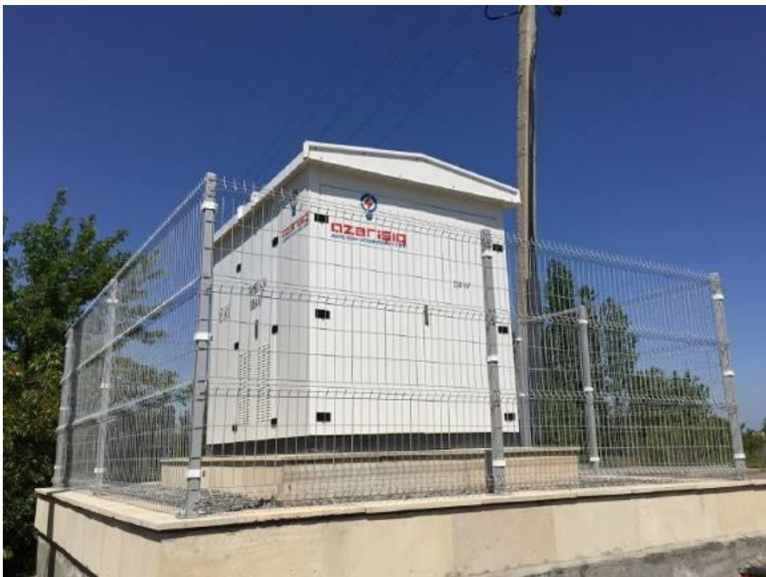
Figure 3: Complete Transformer Substations (CTS)
