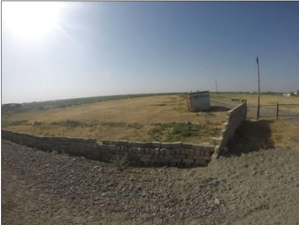
Proposed site for the new Rasullu 35kV substation, Imishli. This site is typical of other sites where new greenfield substations are propose.
