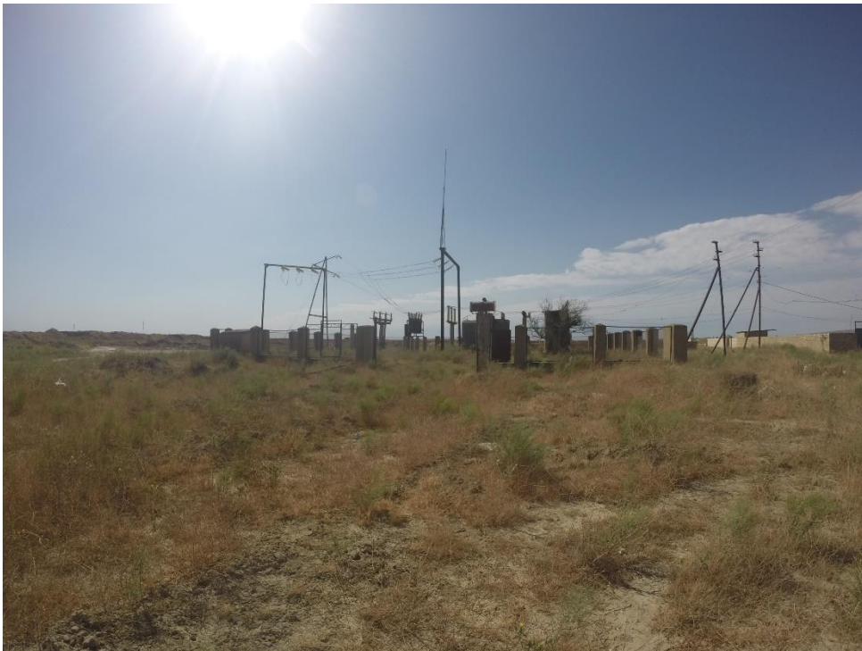
Existing 35 kV Alat Baglar substation that will be replaced within the same site
