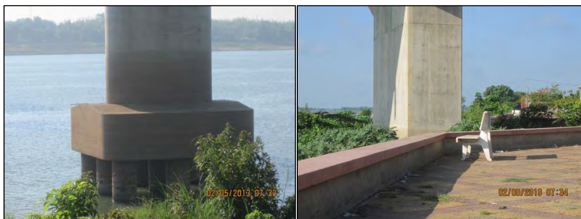
Figure 11 Staining on Bridge Pillars and View of the Parapet (Source: MICO Consultant studies)
