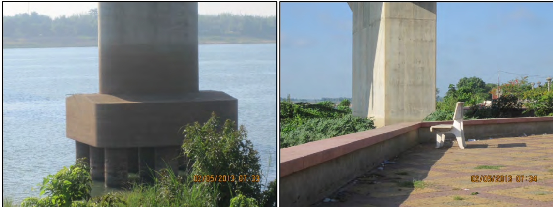
Figure 2 Staining on Bridge Pillars and View of the Parapet (Source: MICO Consultant studies)
