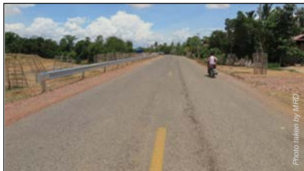
Figure 12: Road section of 1BB1 in Battambang with newly installed road markings
