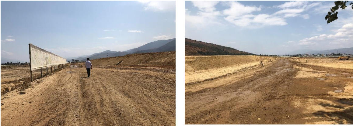
Figure 1-1 site of Xichang Station and project information bulletin board
