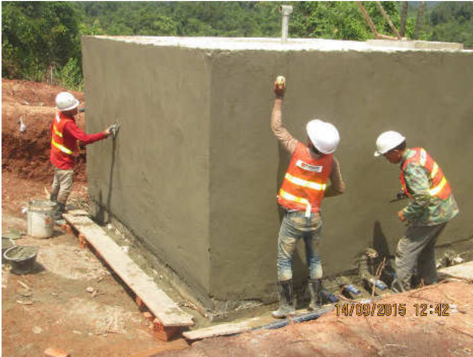
Figure 9 Construction of the water storage tank
