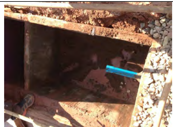
De-oiling pond in the workshop of the Right Tunnelling camp
