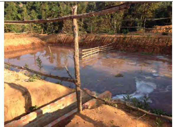
Waste water pond of the Songda Camp
