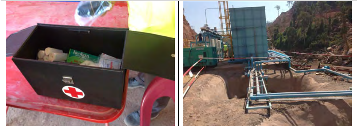
Sanitary kit at the construction site
