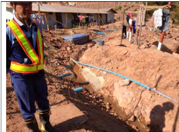
Waste water collection system of the Right Tunnelling camp
