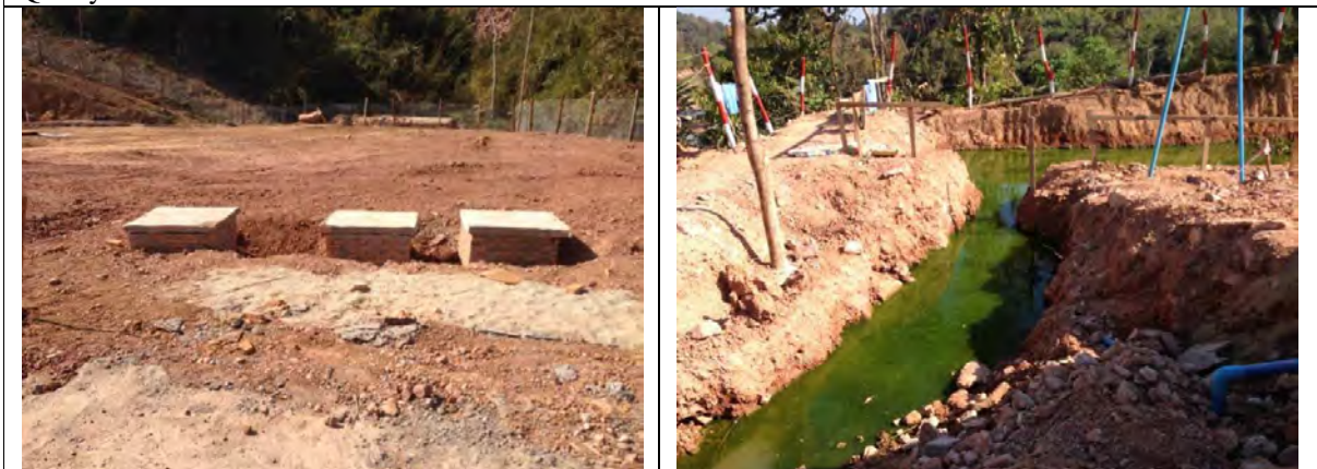
Septic tank of the Sino Hydro Camp
