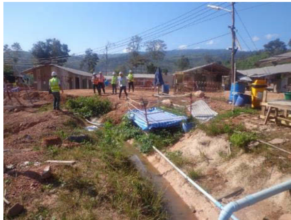
Photo 3: Sediment and Erosion Control Structure at the Road T10/T11
