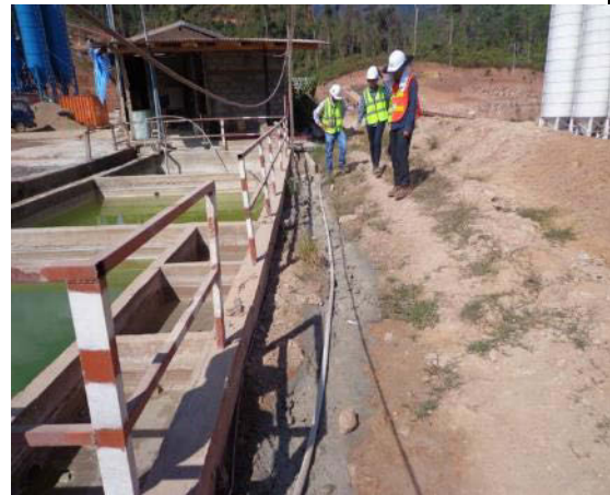
Photo 4 : Improvement of the WWTS of Sinohydro Camp
