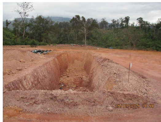
Photo 6: The Fourth Waste Pit
