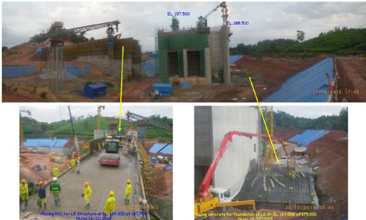
Fig. 3: Status of Re-regulating Dam Works as of December 2015
