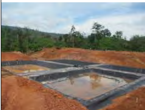
Photograph 6: Completed HDPE lining of treatment ponds
