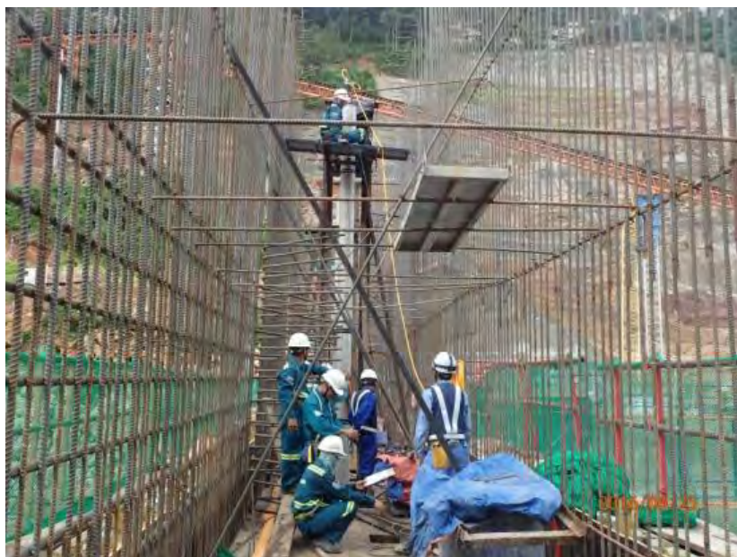
Figure 2-4: Embedded piping installation (Main powerhouse)
