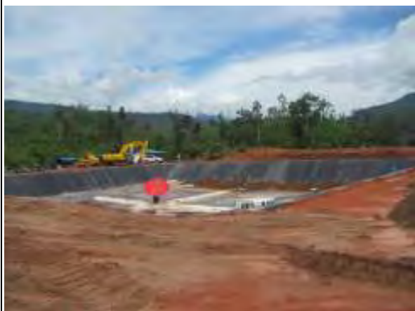
Photograph 5: Completed HDPE lining of sanitary solid waste pit
