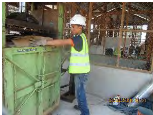
Photograph 14: Installation of the pressing machine
