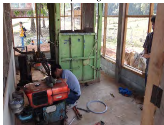
Photograph 14: Installation of the pressing machine
