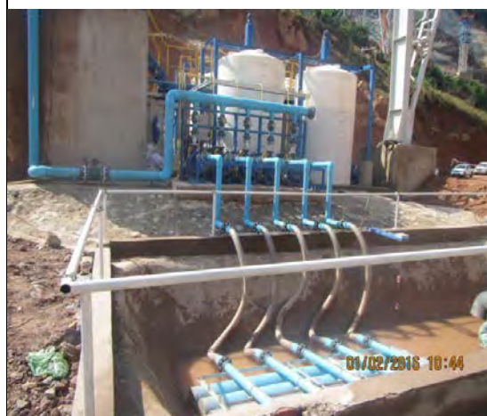
Photograph 4: Joint bi-weekly inspection on the improvement of the WWTs for main dam and powerhouse areas
