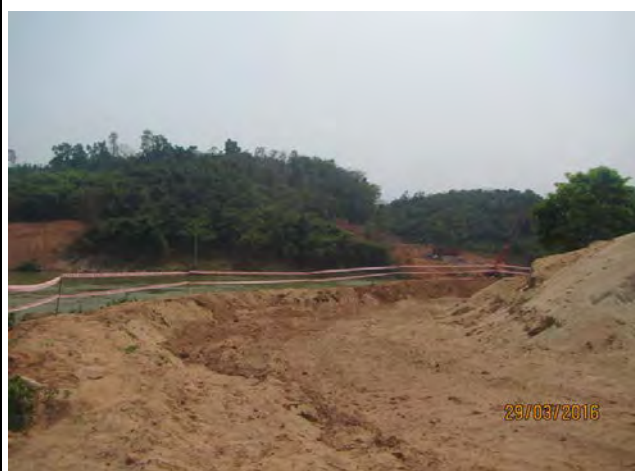
Photograph 3: Weekly follow up inspection on the erosion and sediment control at the temporary sand and aggregate material stockpile yard, Nam Ngiep River on the left bank
