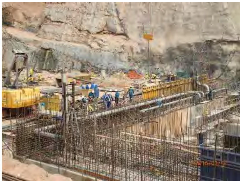
Figure 3-4: Embedded piping installation (Main powerhouse)
