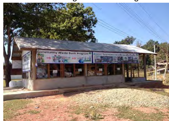
Photograph 13: The extended storage area for ressing machine
