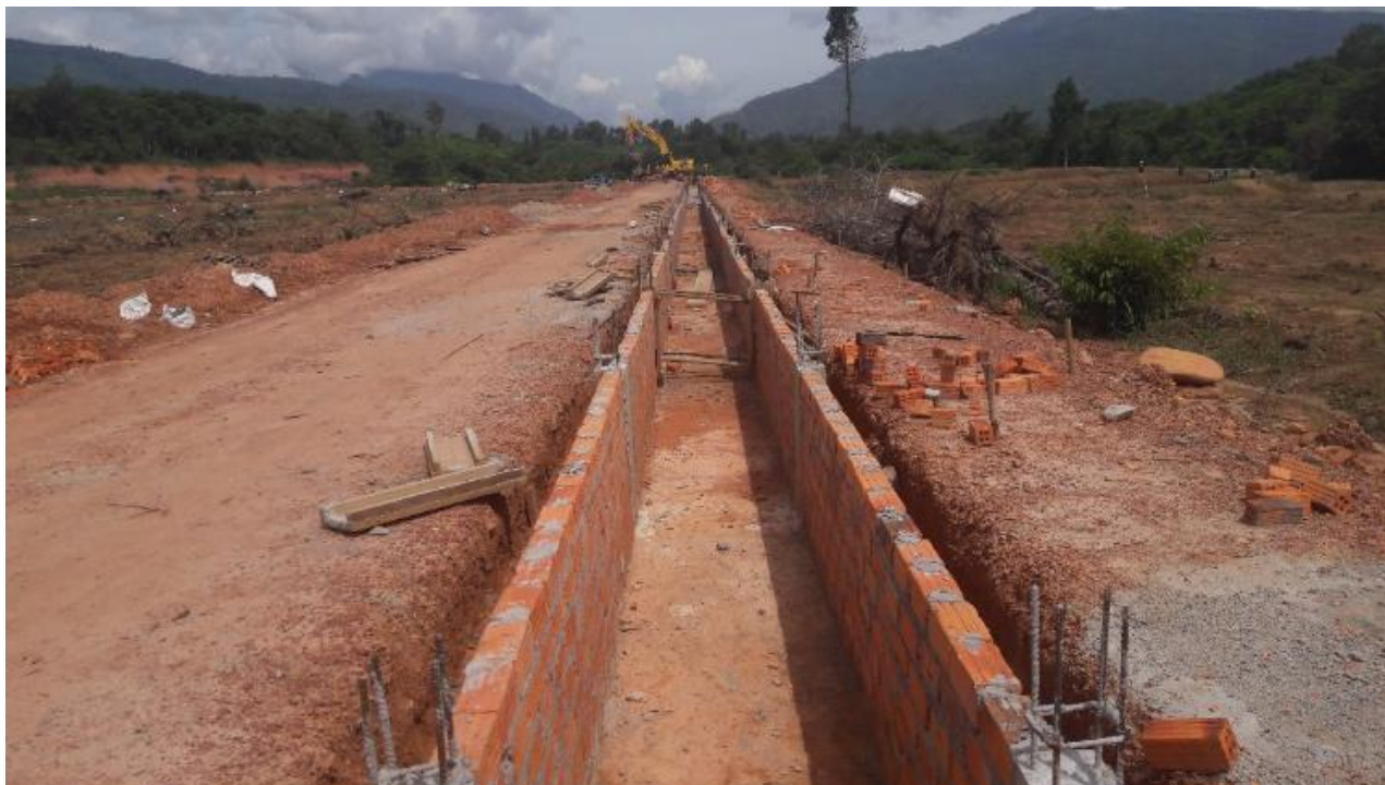
FIGURE 5 PHOTOS SHOWING PROGRESS ON IRRIGATION CONSTRUCTION IN HOUAY SOUP RESETTLEMENT AREA
