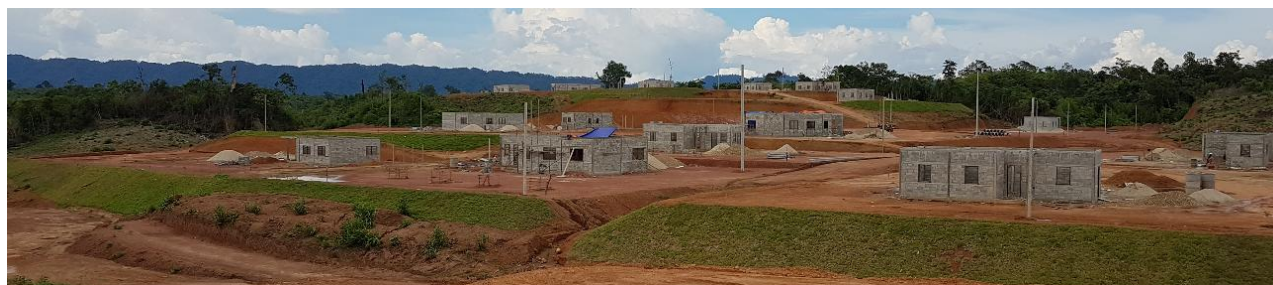
FIGURE 3 PHOTOS OF HOUSE CONSTRUCTION IN HOUAY SOUP AND ITS PROGRESS
