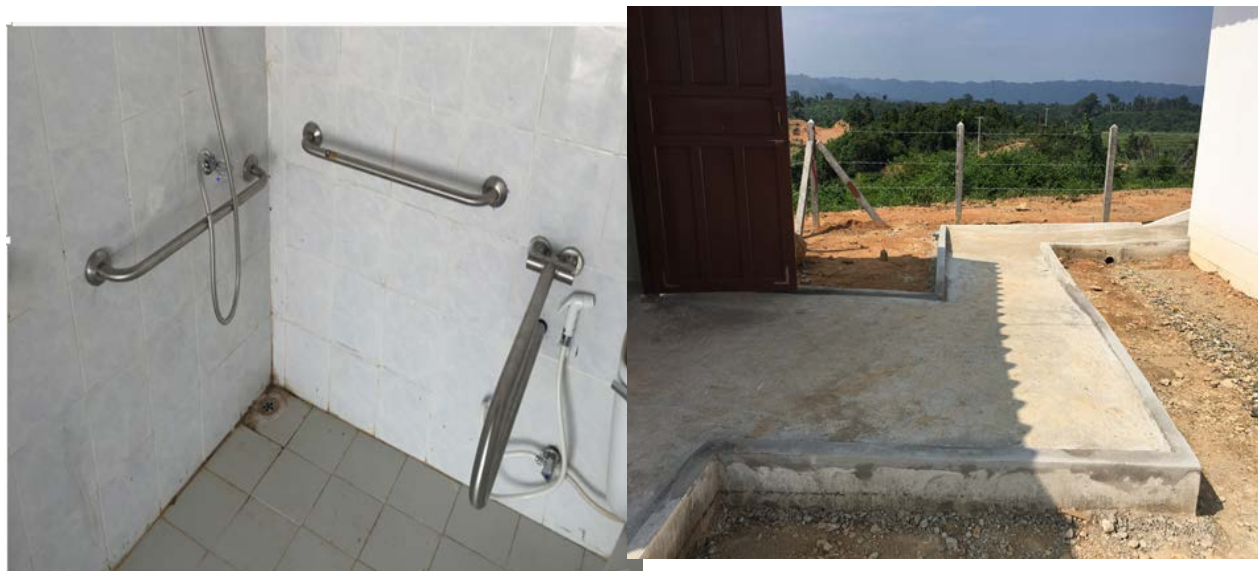
FIGURE 14 MODIFICATIONS MADE TO THE HOUSE FOR USE BY THE PERSON LIVING IN A WHEELCHAIR
