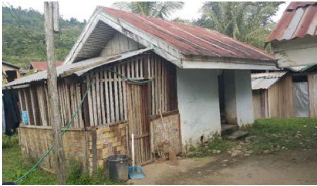
Latrine building (before)
