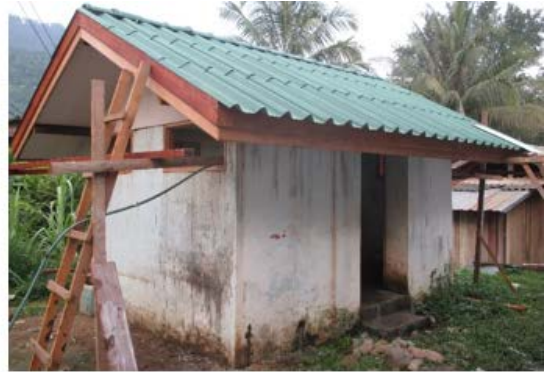
Latrine building (after)
