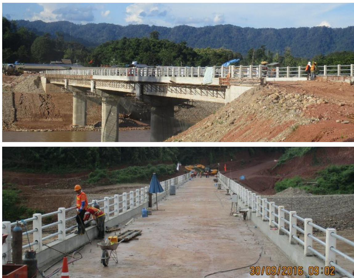
FIGURE 4 PHOTOS OF BRIDGE CONSTRUCTION FOR THE ACCESS ROAD TO THE HSRA
