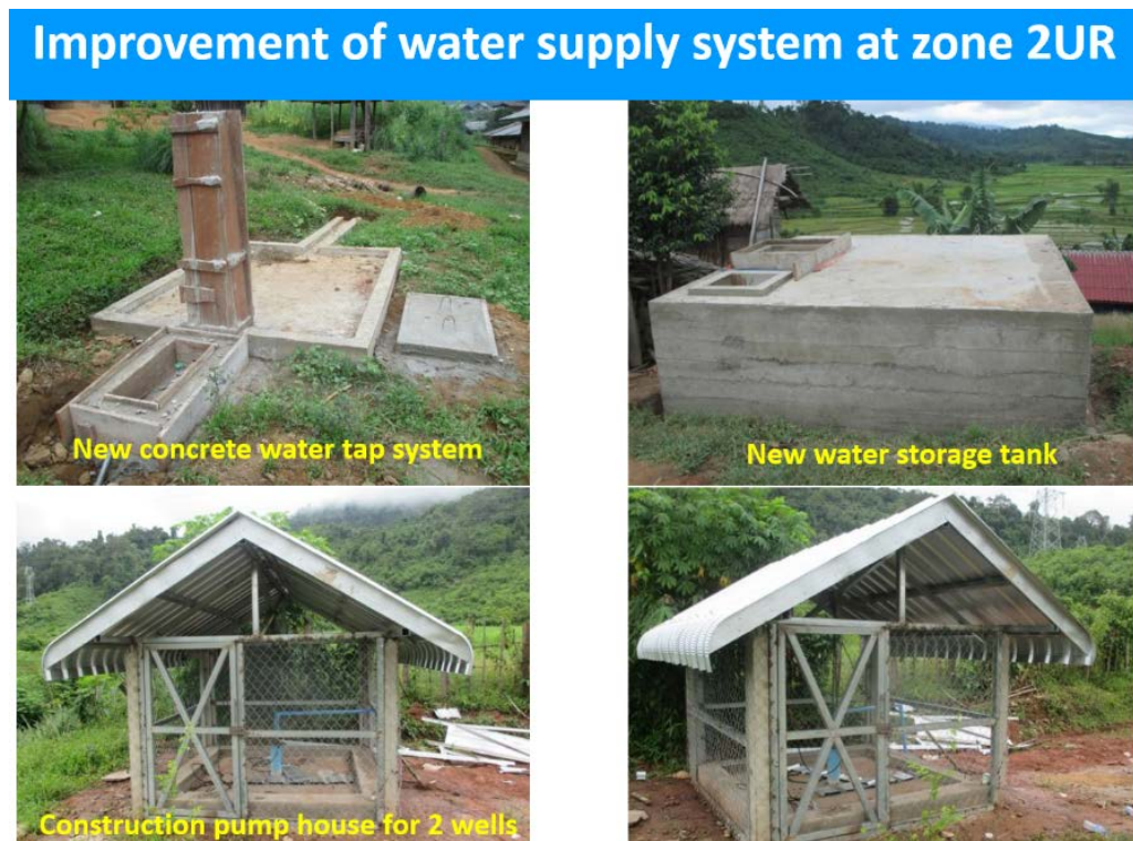
FIGURE 8 PHOTOS SHOWING PROGRESS ON THE IMPROVEMENT OF THE WATER SUPPLY IN ZONE 2UR
