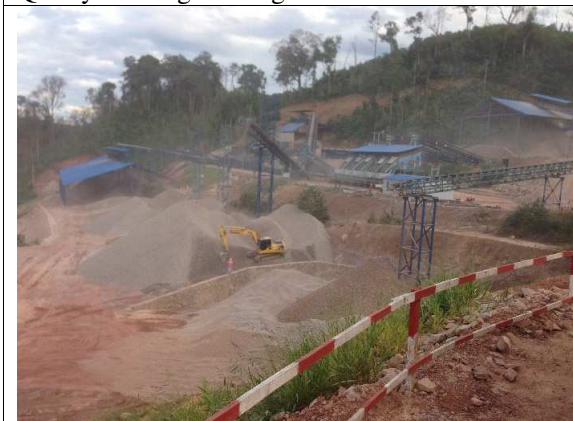
The crushing plant: note the dust
