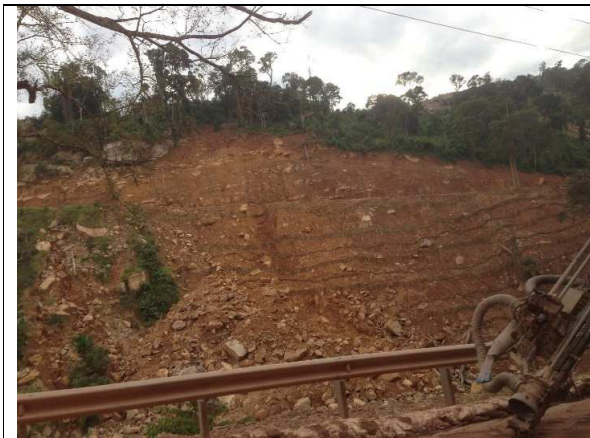
Silt fences downstream the dam axis
