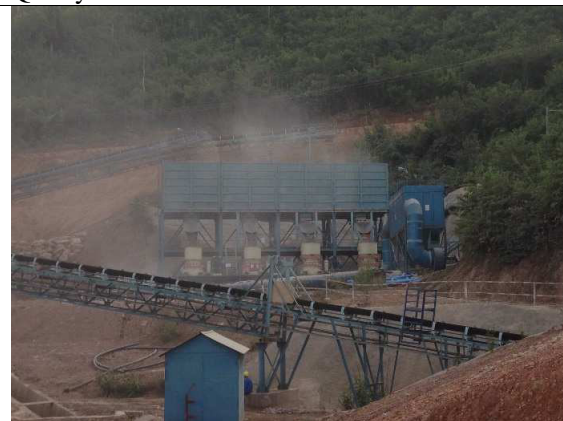
Crushing plant: detail
