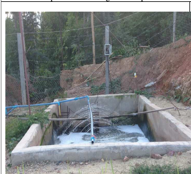
Wastewater treatment pond at Obayashi camp
