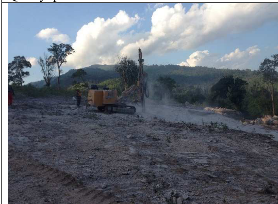
Quarry: drilling blasting holes
