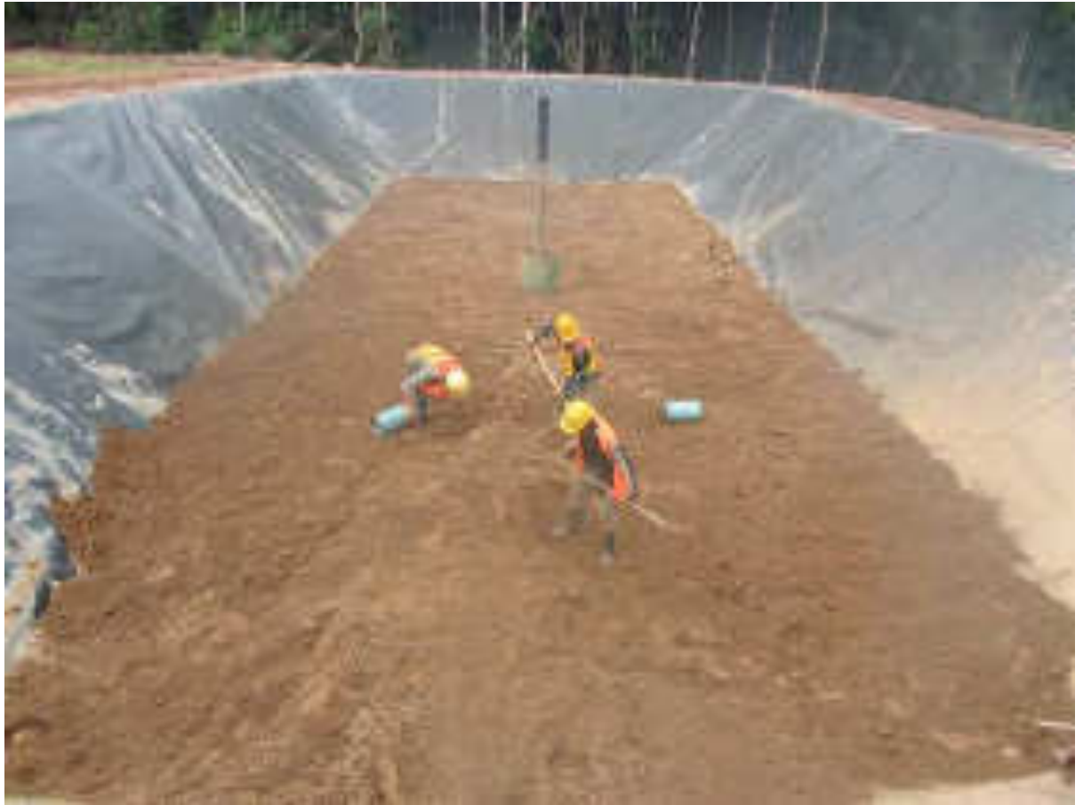
Figure 45 Lined waste disposal pit under construction in the HSRA (Infrastructure development 2016)
