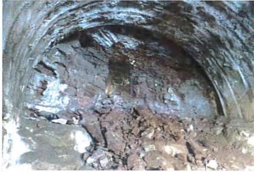
Photo 6: The Breakthrough at the Top Bench on 30 June 2015
