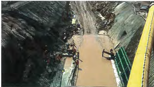
Photo 37: Pooled Effluent Water at the Tunnel Outlet Excavation Site (April, 2015)
