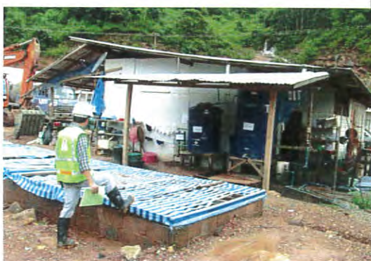
Photo 13: Grey Water Treatment System at the RT Camp Located next to the Kitchen
