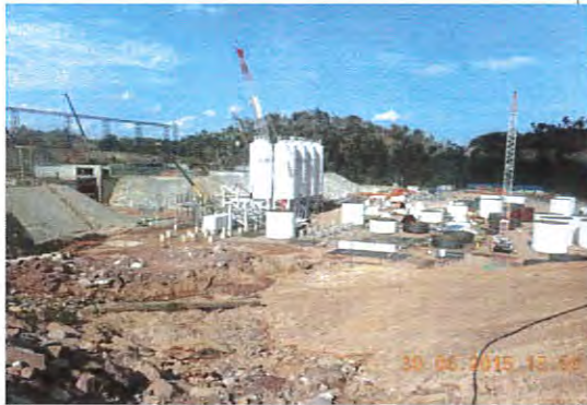
Photo 15: Roller Compacted Concrete plant
