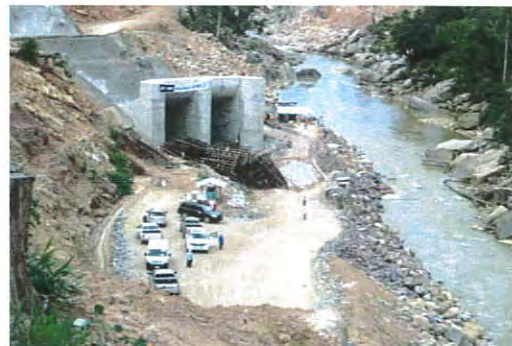
Photo 9: The Inlet Diversion Tunnel
