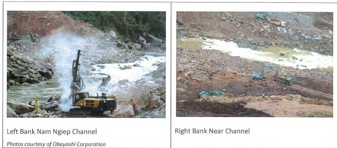
Photo 4 and 5: Main Dam Excavations, June 2015
