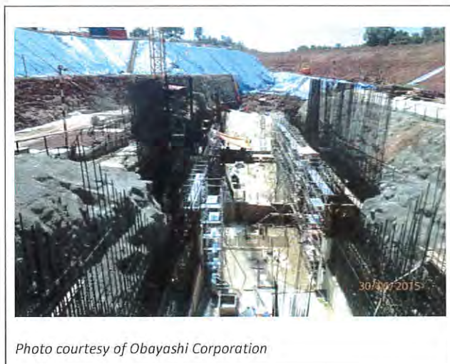
Photo 10: Regulation Excavation (left bank) the background, June
