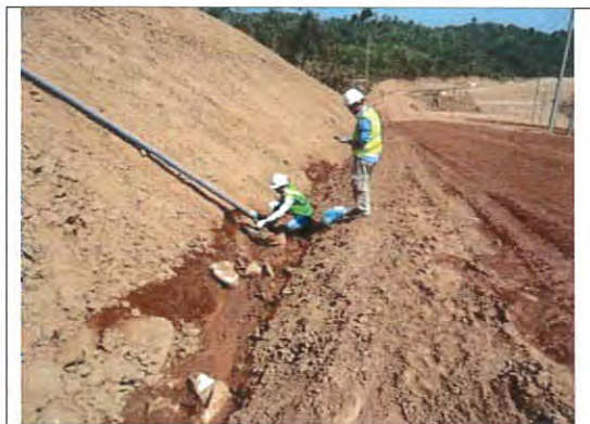
Photo 36: Sinohydro grey water treatment system discharge location
