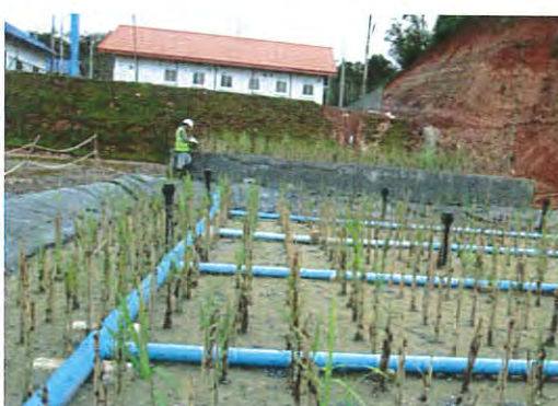
Photo 14: Grey Water Treatment System at the Owner Base Camp
