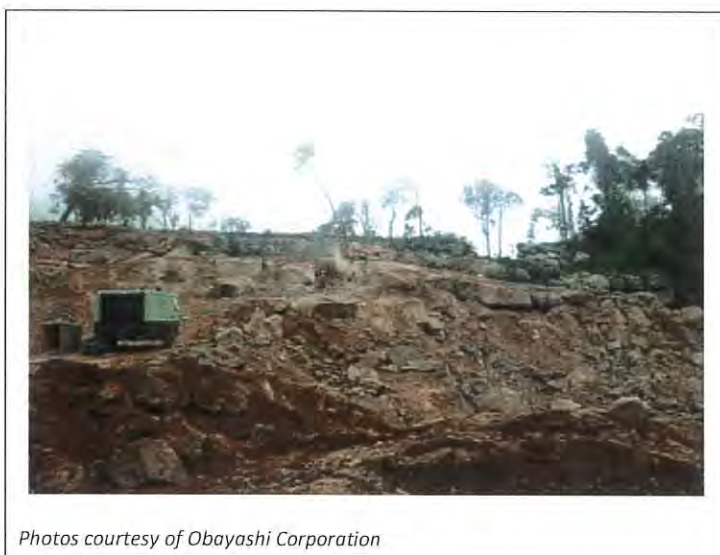
Photo 3: Main Quarry Overburden Removal, June 2015
