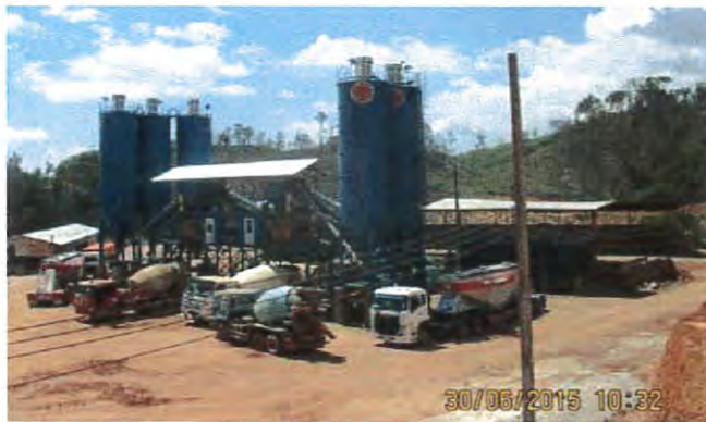
Photo 17: Conventional Vibrating Concrete plant (to right of photo, under construction)
