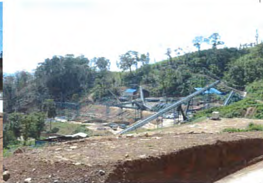
Photo 16: Aggregate Crusher Plant (with conveyor system under assembly), June 2015
