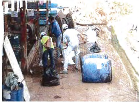
Photo 21: Cleaning up of Hazardous Waste Storage Area after Material Collection
