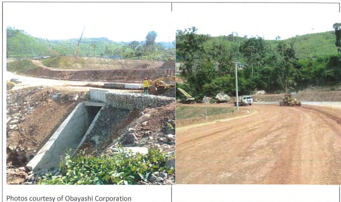
Photo 1 and 2: Completion of Access Roads by June 2015
