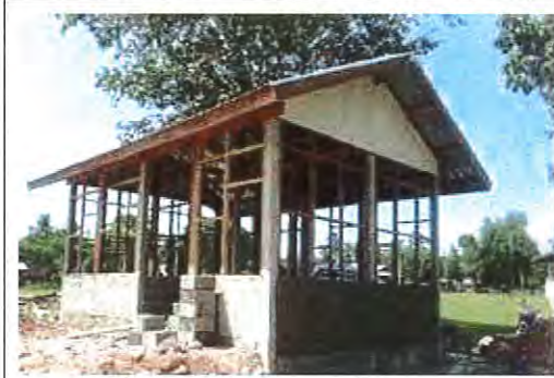
Photo 32: Community Recycle Bank Was Being Constructed
