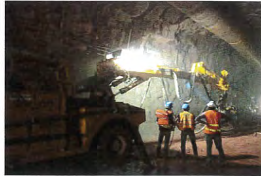
Photo 7: Shotcrete Lining of the Tunnel Wall
