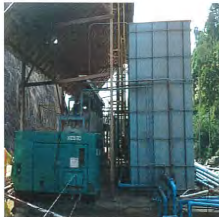
Photo 38: The Effluent Filtration System used at the Tunnel Outlet Excavation Site which is Situated on the Upper Left Bank of the Tunnel Excavations
