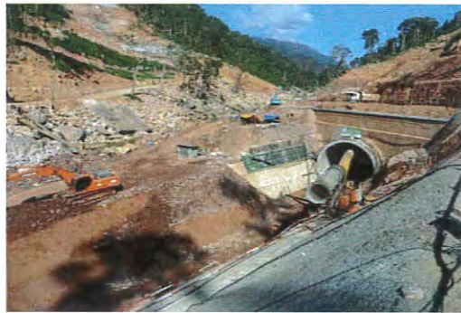
Photo 8: The Outlet Diversion Tunnel
