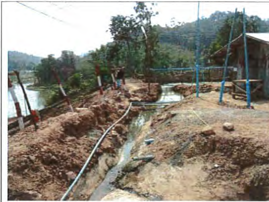
Photo 34: Right Tunnel Grey Water Treatment Pond
