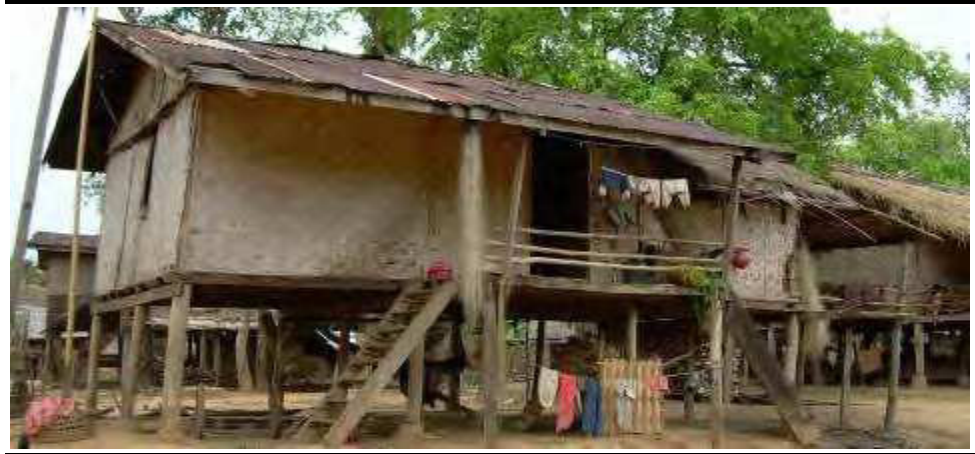
Figure 5.30 Houses at Ban Hat Gniun
