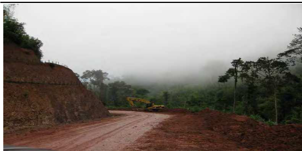
Figure 6.3 Large Sediment Load due to Unpaved Road
