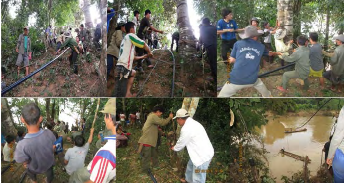
Figure 1: Water Supply Repairs in Sopyouak Following Flood Damages
