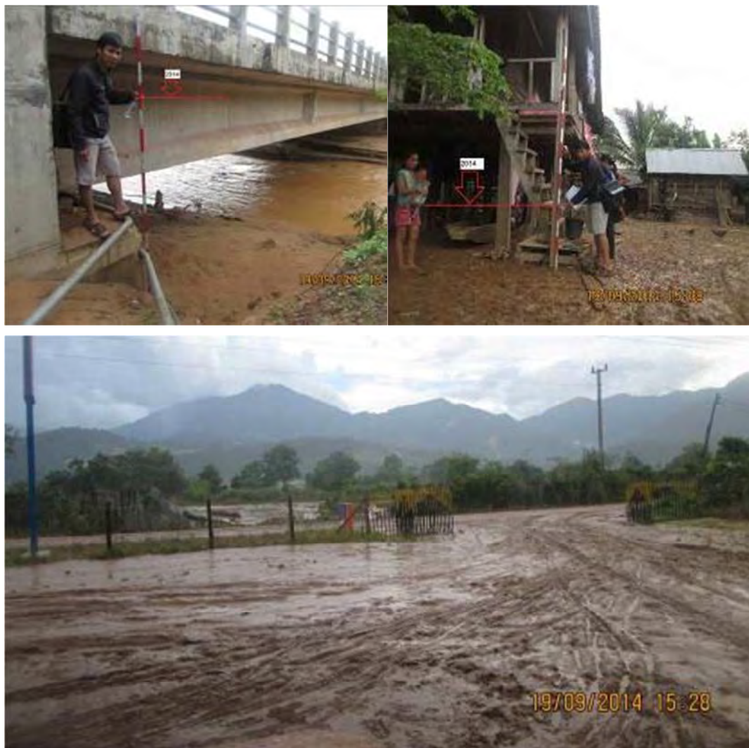
Figure 14: Flooding in Thaviengxay / Thathom District in September 2014
