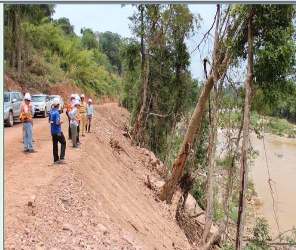
Less attention and investment in mitigation measures is being made by the Contractor to provide erosion control along temporary roads (i.e. lack of drainage and lack of revegetation for slope protection)
