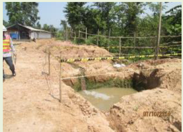
Addressing sewage treatment and waste management issues at camp sites is an important environmental issue of dispute between the EMO and the contractors. This sedimentation pond holds wastewater from the camp but provides inadequate treatment efficiency. Wastewater discharges do not meet Lao effluent standards.
