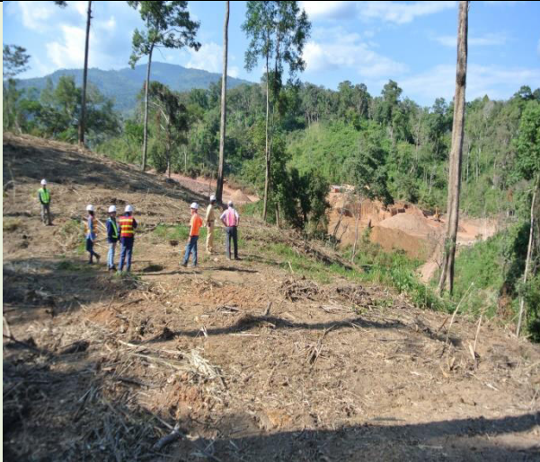
Location of NNP1 landfill during the construction phase. Landfill designed by NNP1 to international standards and will be built and operated by Obayashi. All construction wastes will be collected, recyclable materials separated, and wastes disposed of at this site from all contractors and NNP1. Service fees will be calculated and agreed upon prior to start-up.
