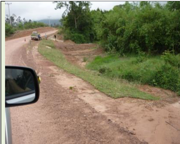
Re-vegetation of selected areas along permanent road during the current dry season to minimize future erosion control
