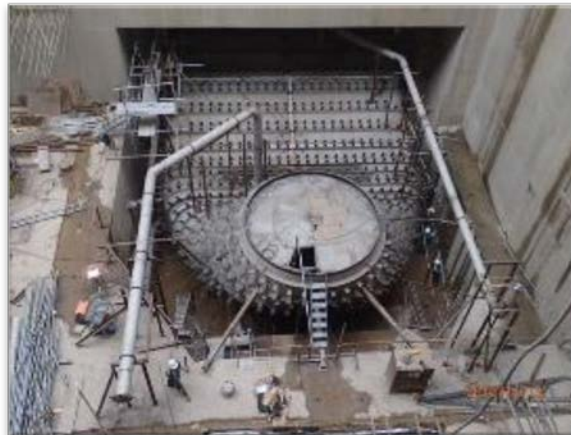
Figure 3-8: Installation of Draft Tube for 1 at the Main Powerhouse
