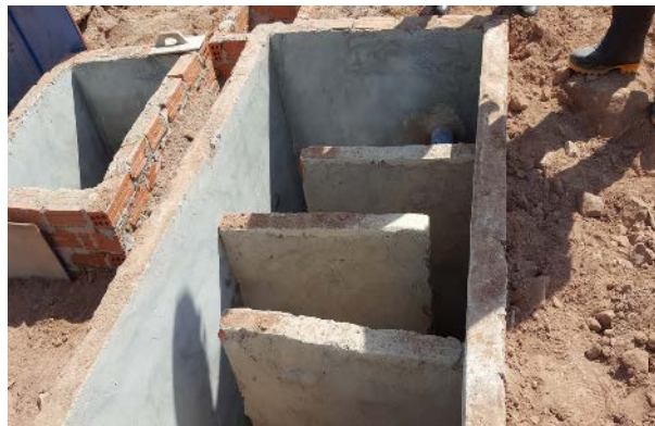
Photo 1: Chlorine Contact Tank at Song Da5 Camp No. 2 in November 2016
