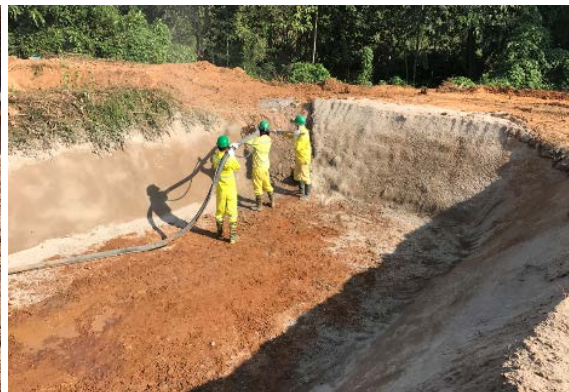
Photo 2: Progress of the WWTS Improvement at Song Da5 Camp No. 1 in November 2016
