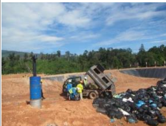
Photo 6: Waste Disposal Spot Checking by NNP1PC staff at NNP1 Project landfill
