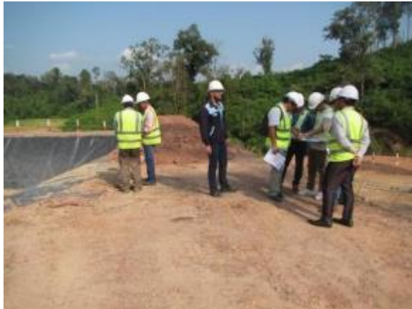
Photo 89: A final inspection of the 1 st stage Houay Soup Landfill construction
