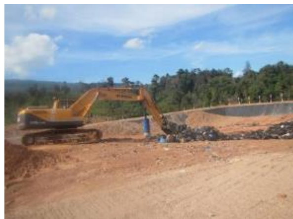
Photo 5: Waste Compaction and Soil Cover at the NNP1 Project Landfill
