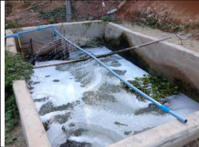
Combined wastewater “aeration” tank at Main Contractor’s Camp. This tank is not adequate to be considered as an aeration tank; there is no separation of solids after the aeration process; effluent from this tank is released to the environment without meeting Lao Effluent Standards.
