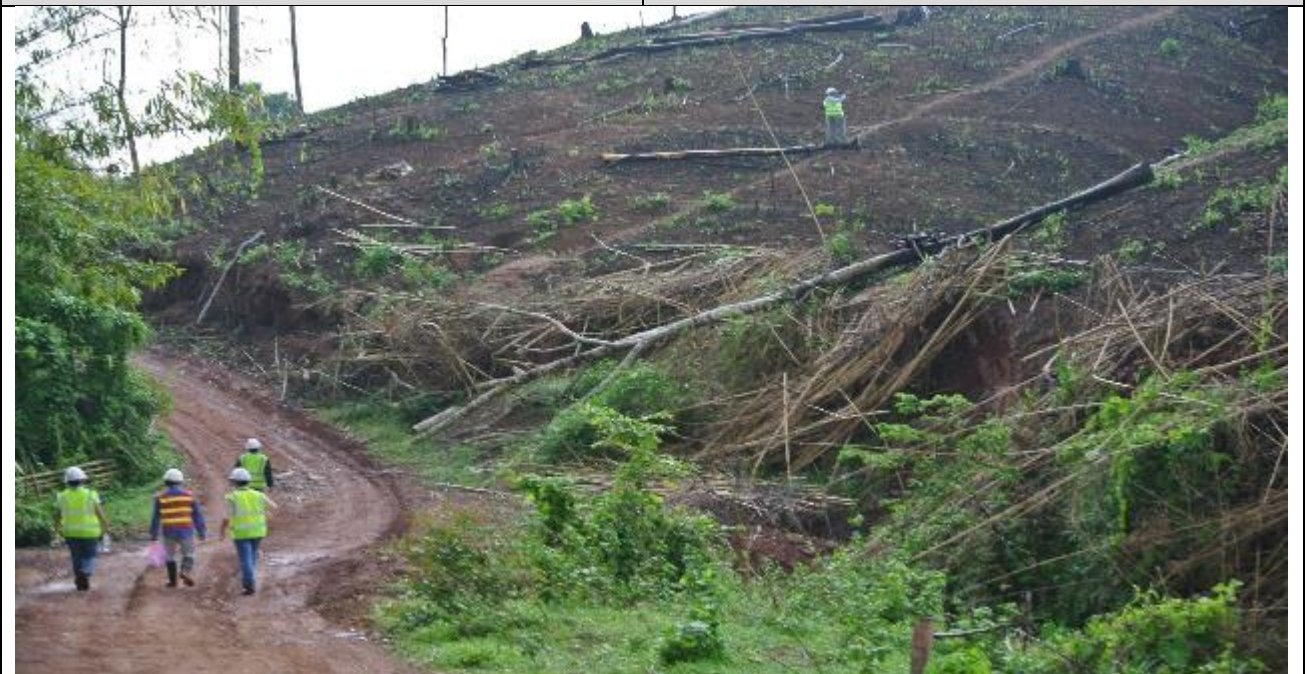
Start of biomass removal in the reservoir area, Block 4, Ban SopYyouak, Hom District. A total of 1,912 ha, divided into 18 blocks, will be cleared of biomass (cut, burn and remove). Local villagers interested to serve as labor register with Village Chief, a contract is signed between villagers and Contractor, villagers are trained and provided with safety equipment, and supervised by contractor’s staff. Cut biomass can be kept and used by villagers for firewood, building huts and re-burn. Villagers can request to use cleared areas for short-term crop plantations.
